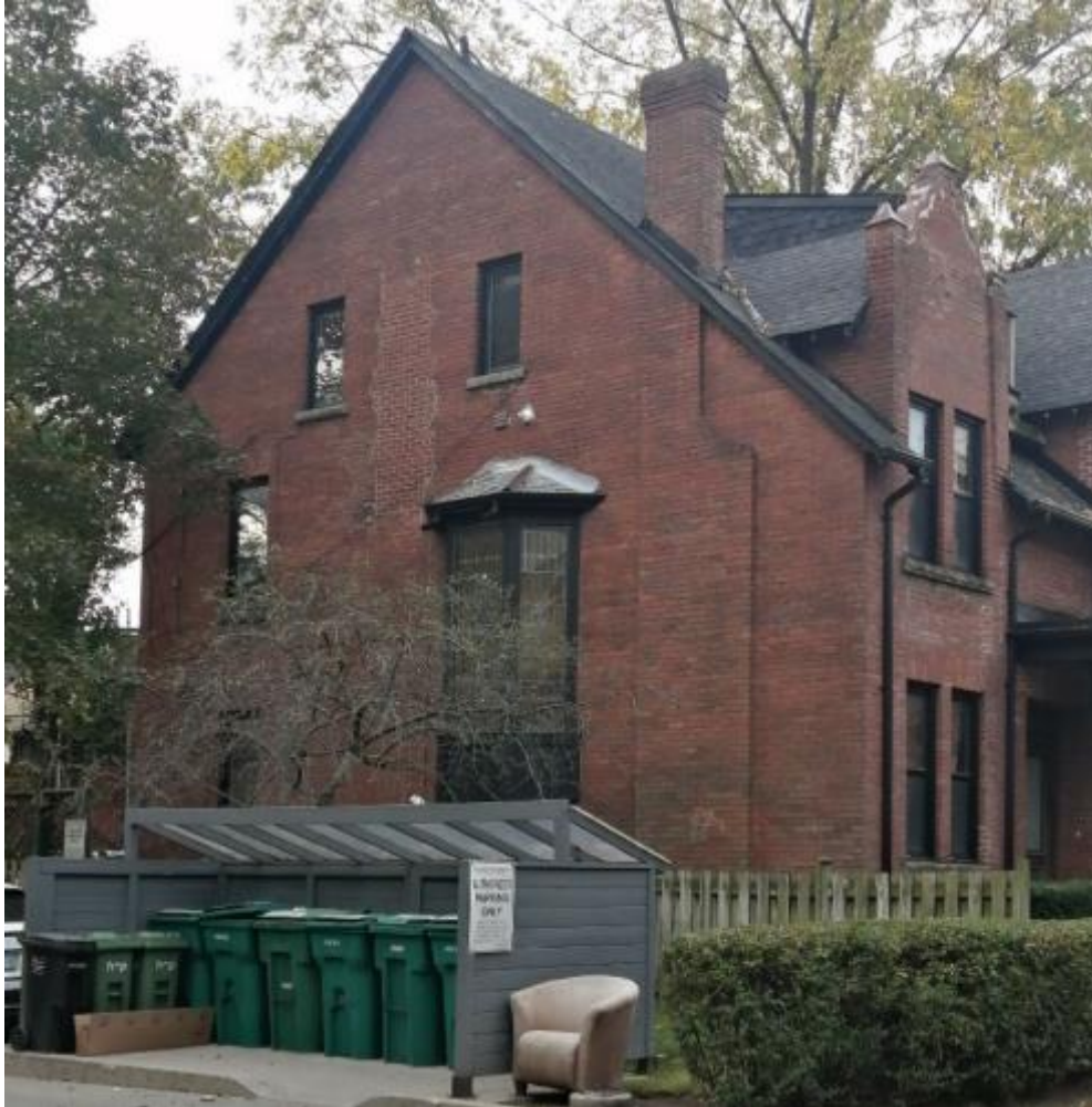
East Elevation (Heritage Planning, 2023)
