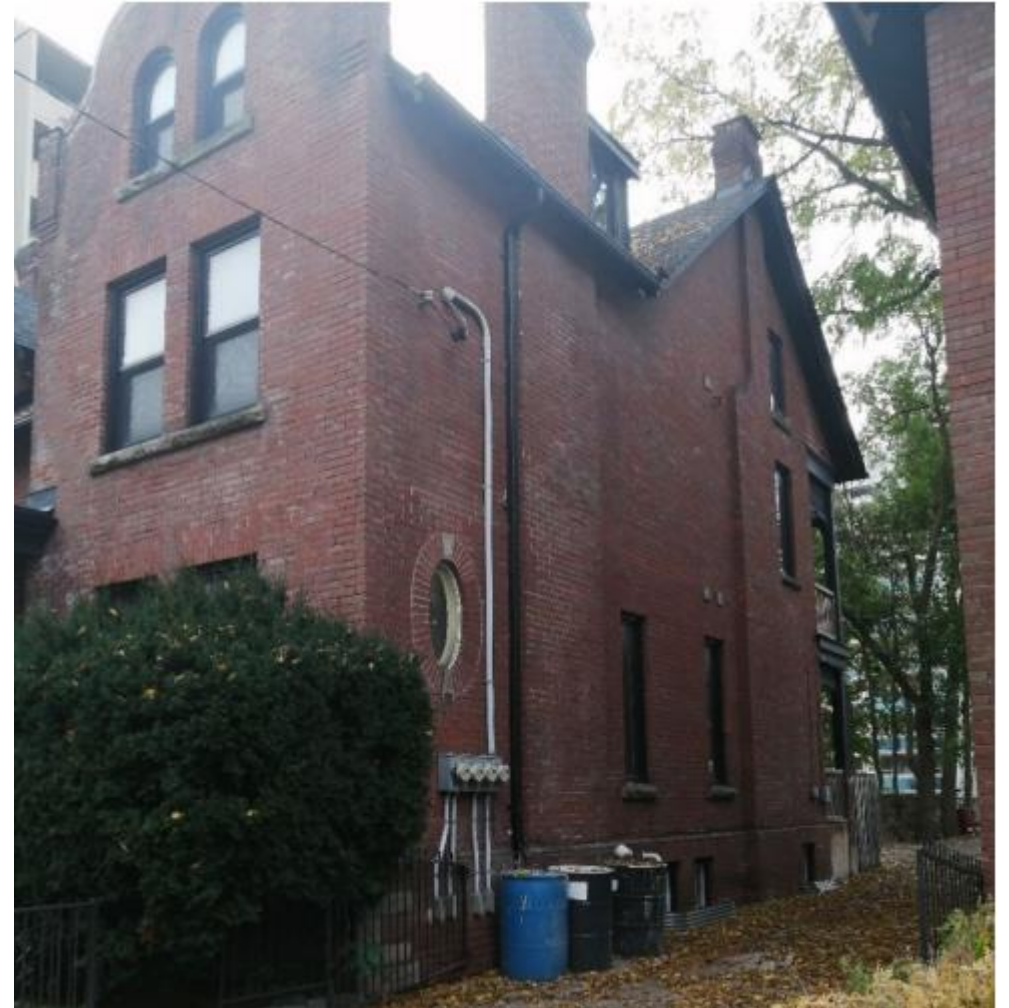
West Elevation (Heritage Planning, 2023)
