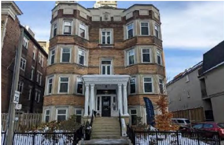
36 (top) & 42 (bottom) Maitland St
