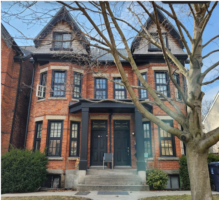
50 and 52 River Street, Heritage Planning, 2024
