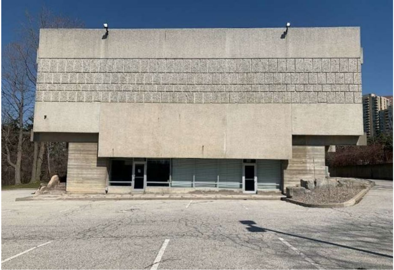
South elevation showing a precast concrete clad building element enclosing the existing backstage, supported on cantilevered beams (Heritage Planning)
