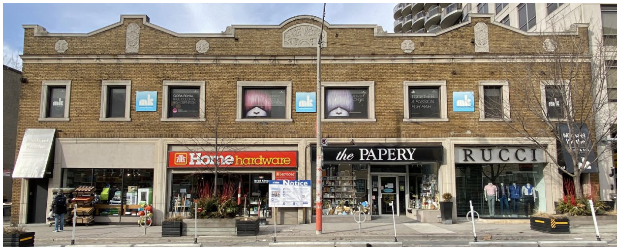
East (primary) elevation of the main street commercial row at 1420 Yonge Street that is now proposed to be demolished (Heritage Planning, 2022)
