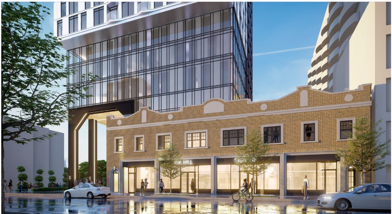
Renderings of the view of approved development illustrating the base of the tower at 1420 Yonge Street that is now proposed to be demolished. (IBI Group)
