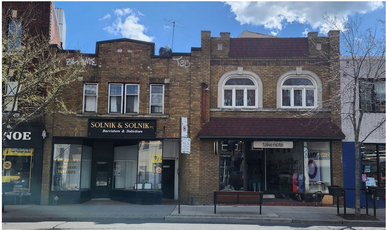
2991 and 2993 Dundas Street West, Heritage Planning, 2024
