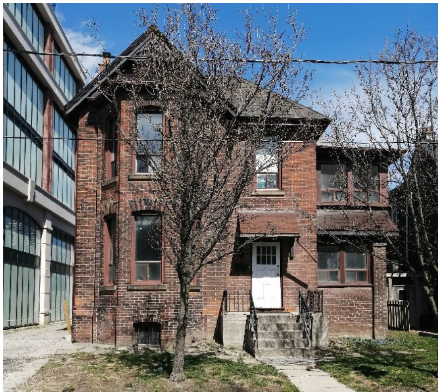
South elevation at 26 Millwood Road (Heritage Planning, 2024).
