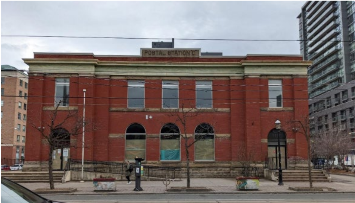
Principal (north) Elevation with two flanking entrances raised above grade and accessed by wide stairways with landings (Heritage Planning, 2022)
