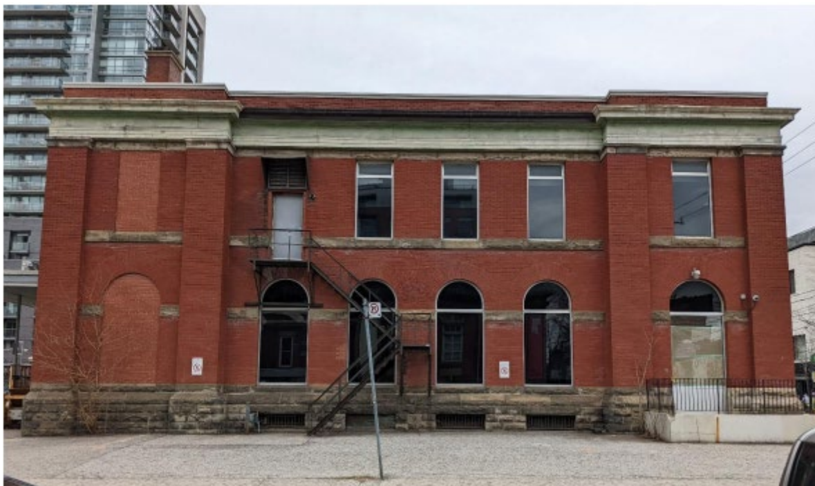
East Elevation (Heritage Planning, 2022)
