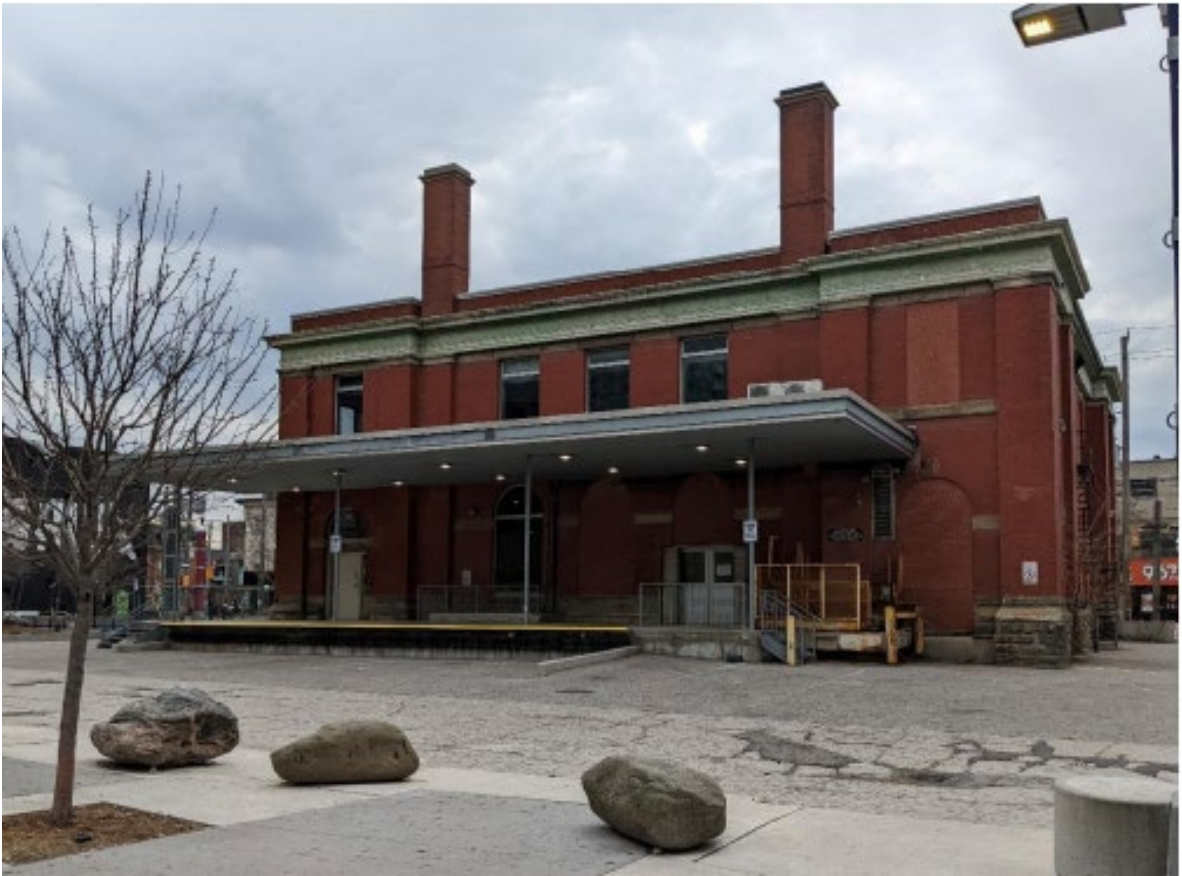
Rear (south) Elevation with loading dock addition (Heritage Planning, 2022)
