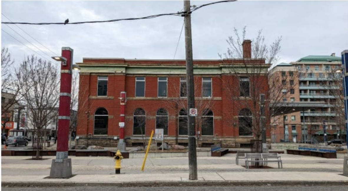
West Elevation (Heritage Planning, 2022)
