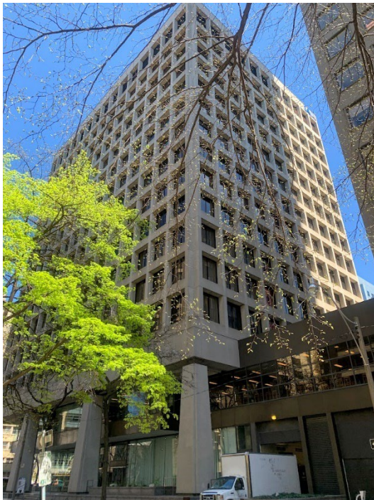
Images 18 and 19: Current photograph of the south and west elevations from Simcoe Street (left); detail of the precast concrete panels and deeply recessed, punched window openings (right). (Heritage Planning, 2024)
