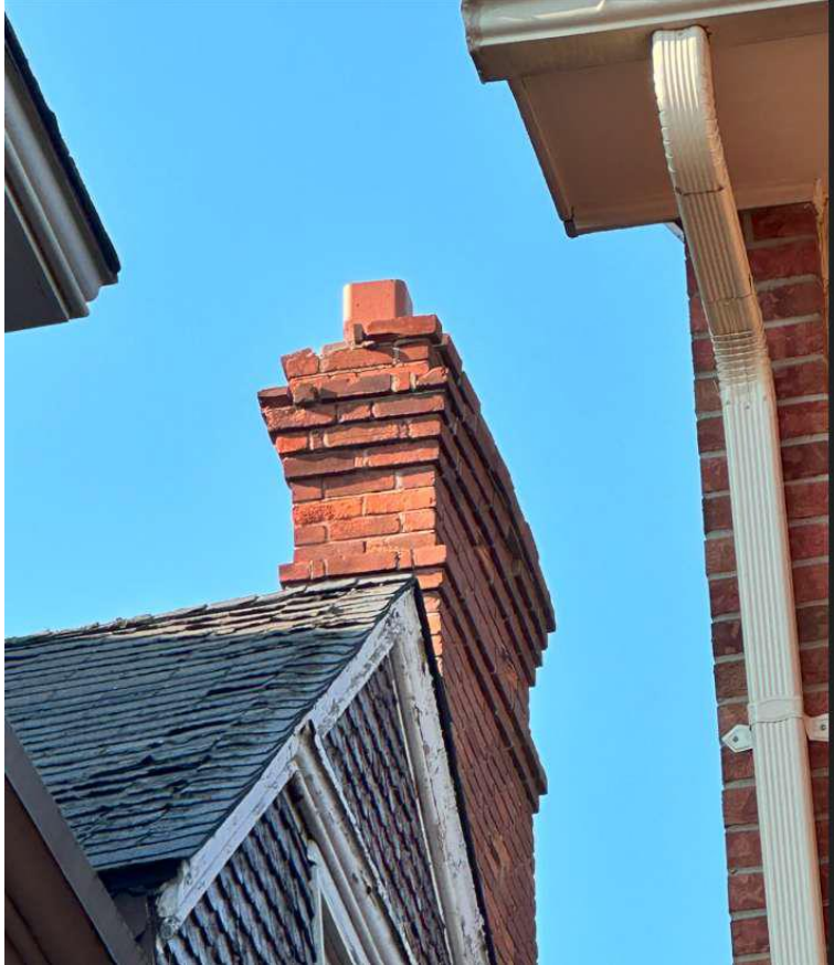
288 Annette Street– Part IV Chimney and roof restoration Grant amount: $7,500
