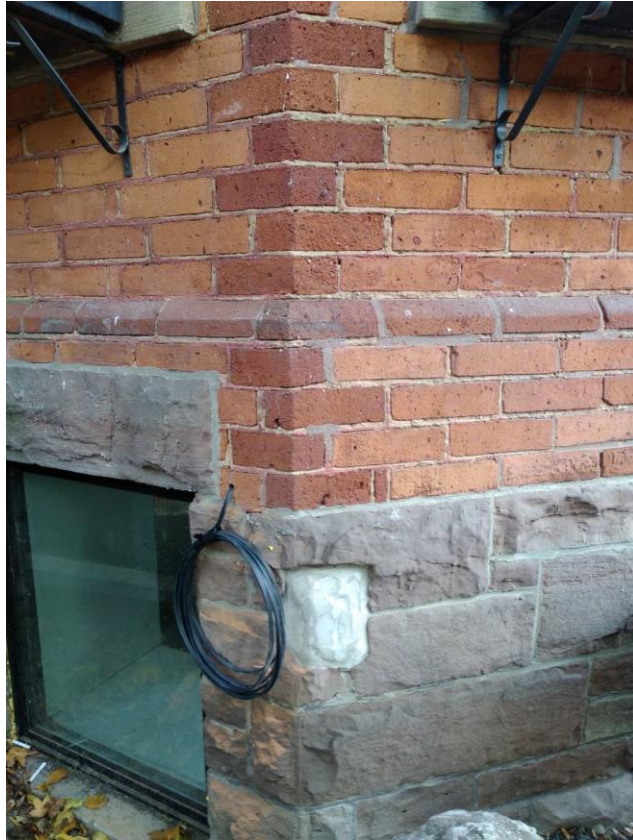
69 Pembroke Street – Garden District HCD Small scale masonry repair and restoration Grant amount: $10,000
