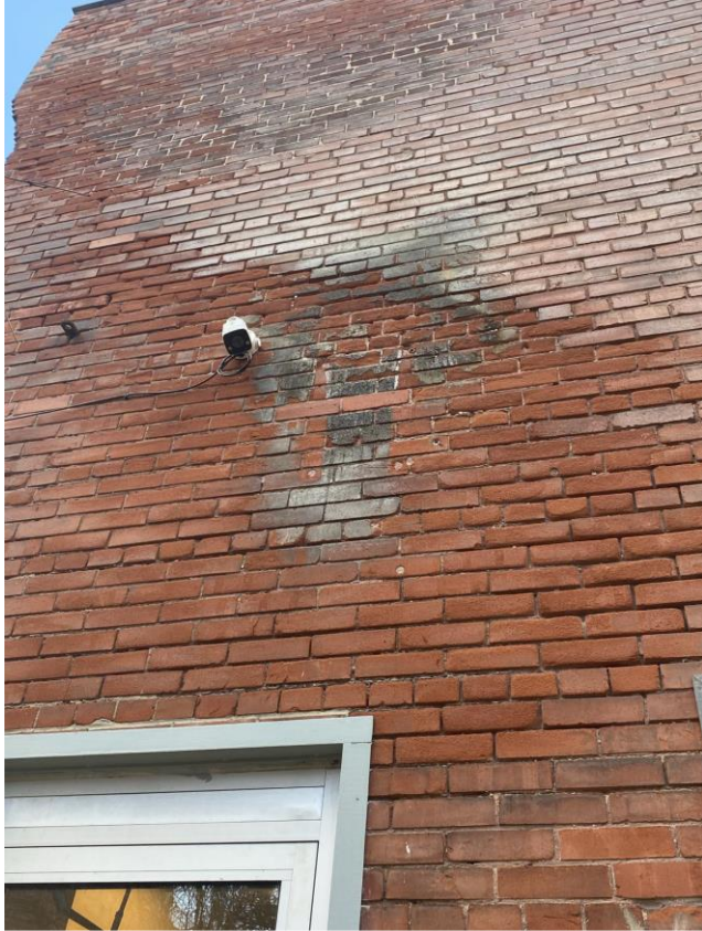
550 Bayview Avenue – Part IV Designation Large scale masonry repair and restoration Grant amount: $110,000
