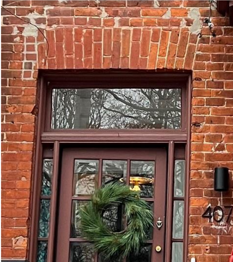
407 Carlton Street – Cabbagetown North HCD Small scale masonry repair and tuckpointing Grant amount: $8,000
