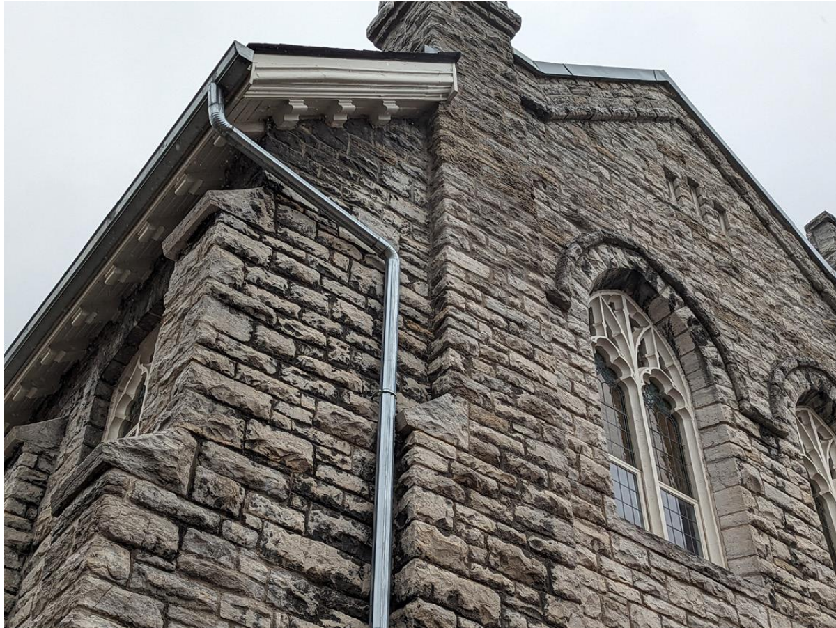
384 Sunnyside Avenue – Part IV Designation Masonry cleaning and wood restoration Grant amount: $20,000
