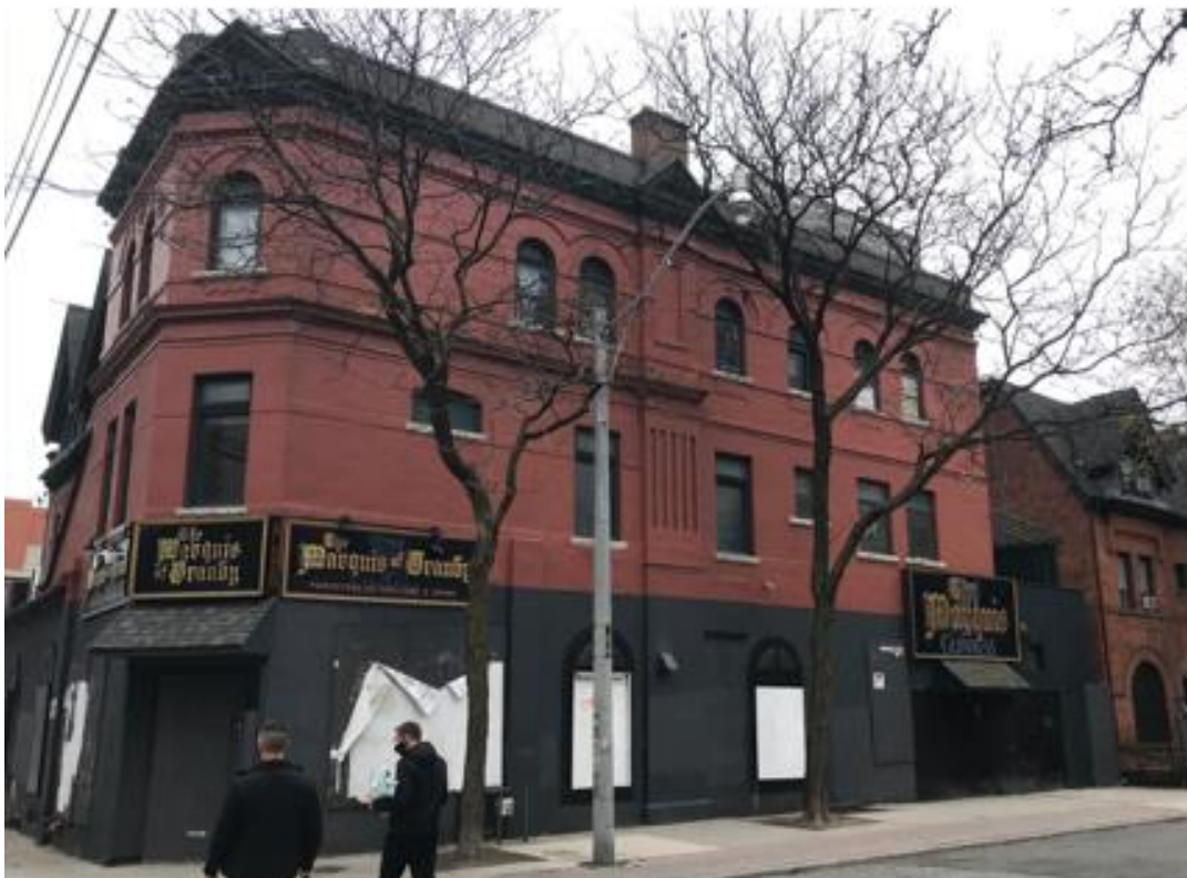
418 Church Street - north (Granby St.) elevation
