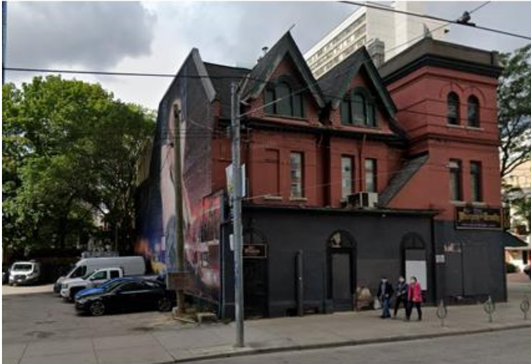
414-418 Church Street - east (Church St.) elevation
