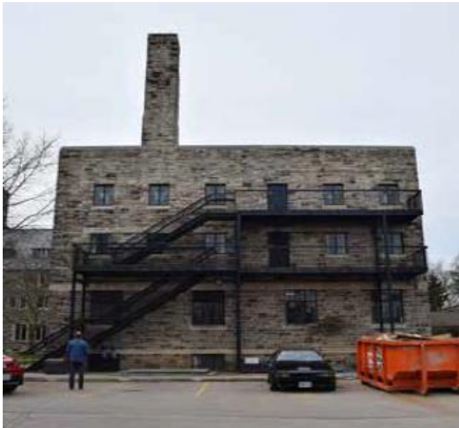
Figure 9. View of the rear (east) elevation of the Convent (north) Wing with fire escape (ERA Architects Inc., May 2022).
