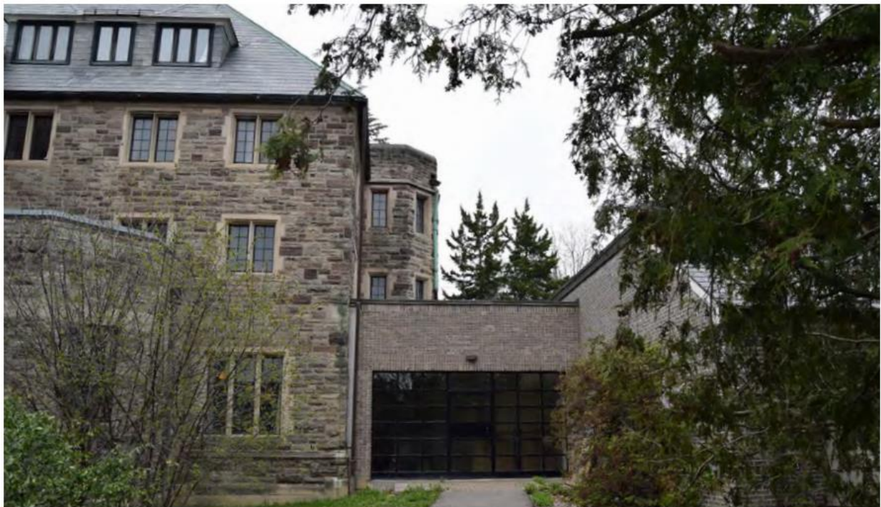
Figure 6. Partial view of the east elevation of the Convent (north) Wing, looking west, showing the one-storey connection with the infirmary (ERA Architects Inc., May 2022).
