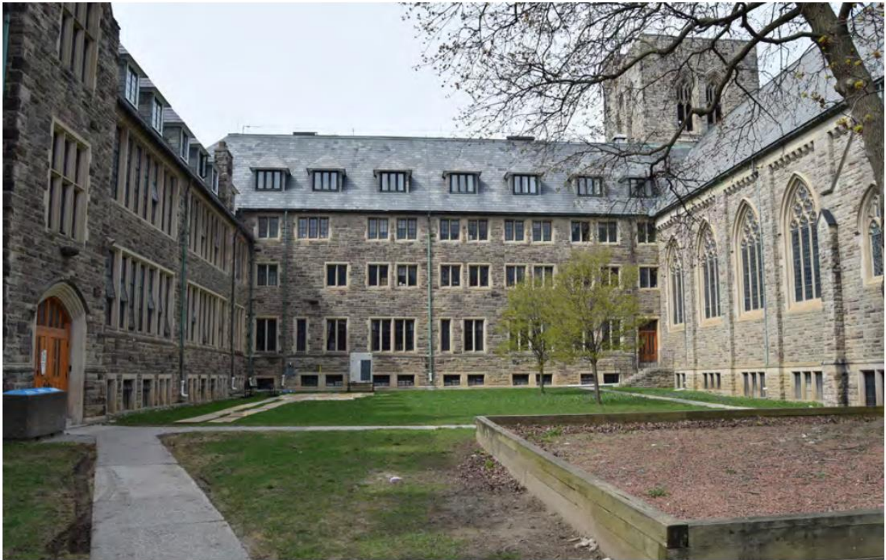
Figure 5. Partial view of the east elevation of the building (showing the School Wing and Chapel) looking west (ERA Architects Inc., May 2022).
