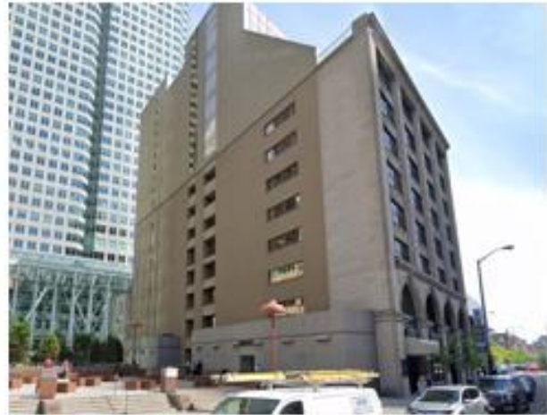
View of west elevation (left)
