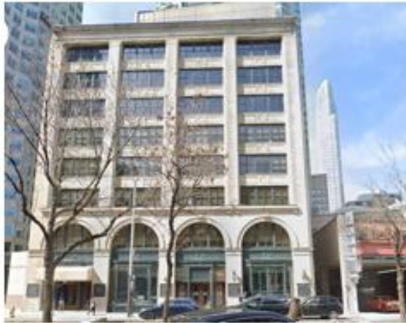
View of south (primary elevation)
