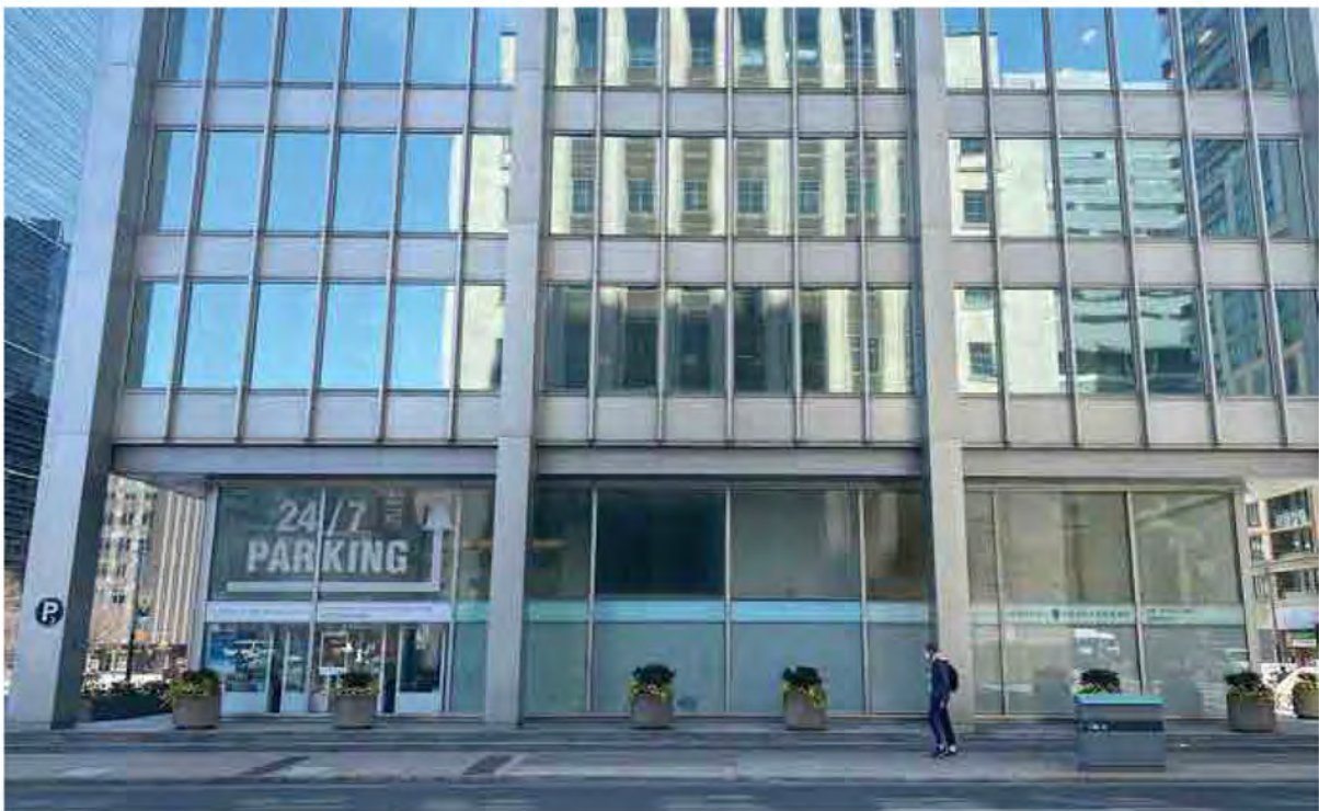
North elevation showing the glass-clad ground floor and mezzanine set back from the building facade (ERA, 2022)
