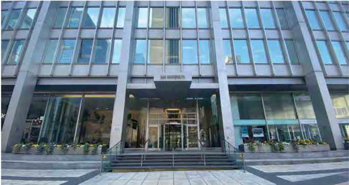
East elevation showing the glass-clad ground floor and mezzanine set back from the building facade (ERA, 2022)
