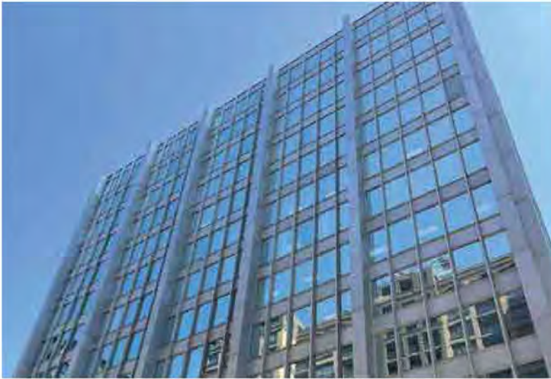
Existing curtain wall and cladding above grade (ERA, 2022).
