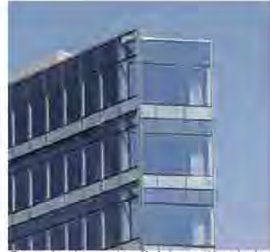
Grey shade, matte finish, unitized aluminum curtain wall with deep extruded caps, and a 5% silver mirrored tint to further differentiate new from existing. (KPMB, 2024)
