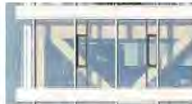
Visible interior perimeter truss visible from exterior creates a horizontal band to transition new from existing (KPMB, 2024)
