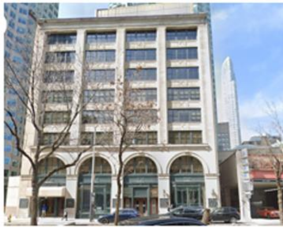
View of south (primary elevation)
