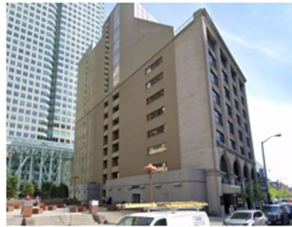
View of west elevation (left)
