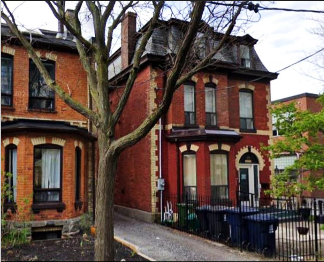
An unobstructed view of 29 Linden Street
