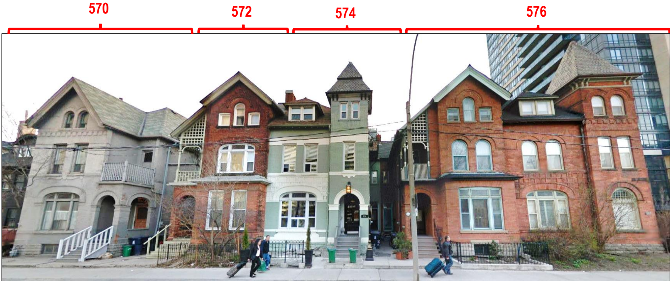
An unobstructed view of 570, 572, 574, and 576 Sherbourne Street
