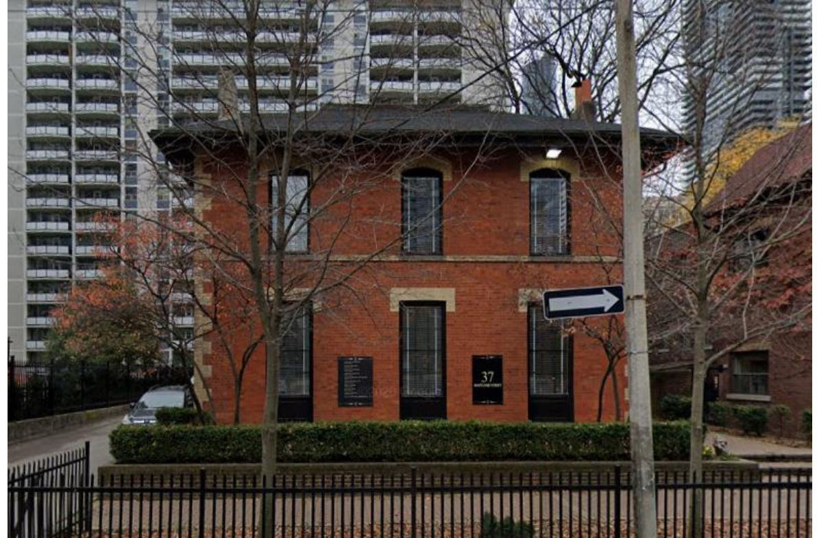
Front (north) elevation of 37 Maitland Street (Google Maps, 2020)
