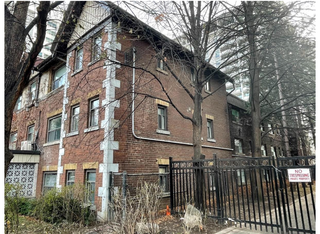
Front (north) and west elevations of 33 Maitland Street (Heritage Planning, 2023)
