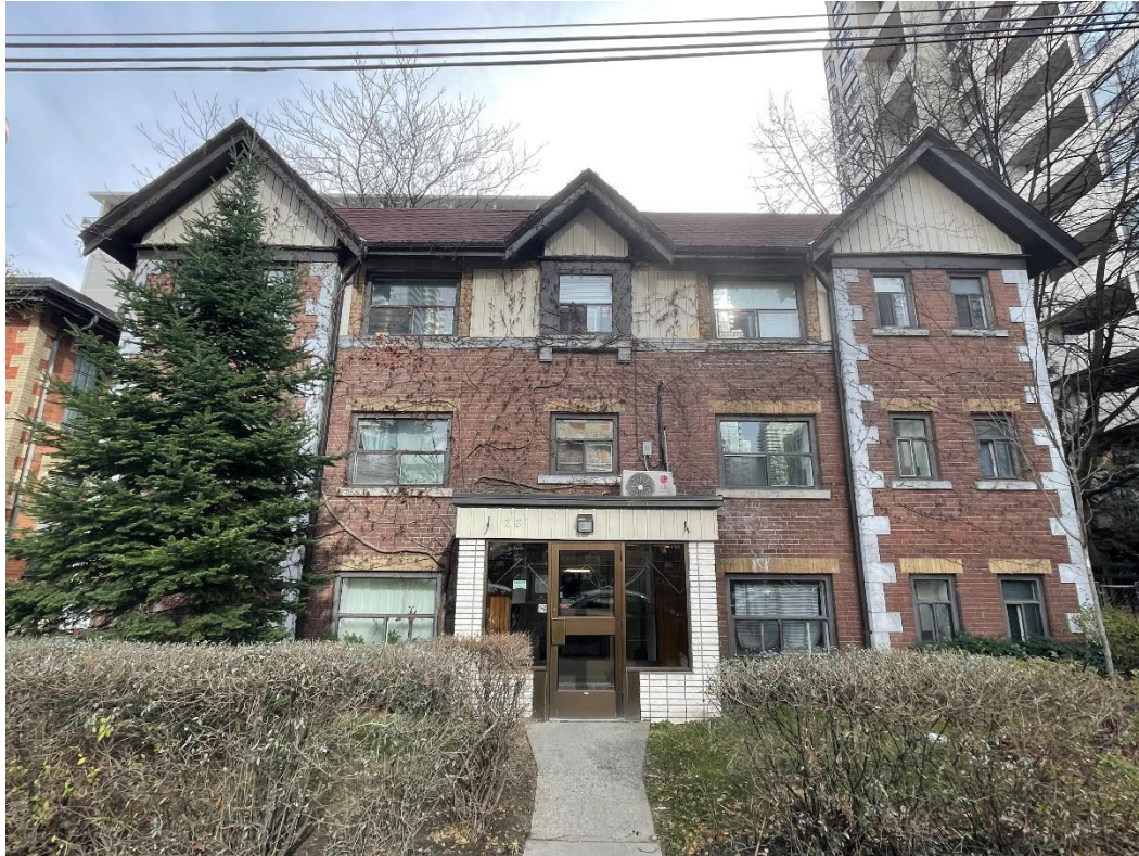
Front (north) elevation of 33 Maitland Street (Heritage Planning, 2023)
