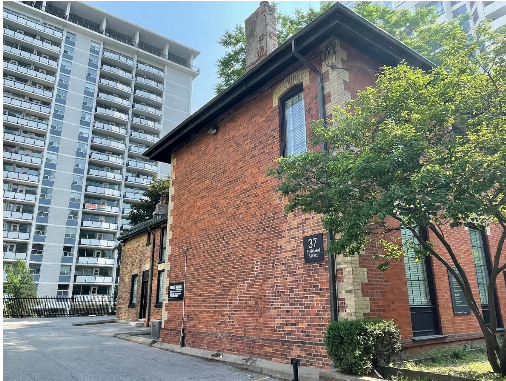
East elevation of 37 Maitland Street (City of Toronto Heritage Planning)(Heritage Planning, 2023)
