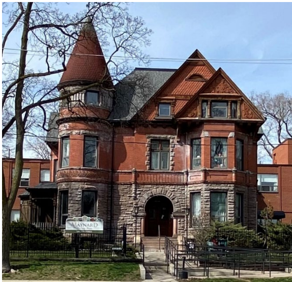
7. The south or principal elevation of 28 Halton Street: elements of the Richardsonian Romanesque style include the heavy massing, rusticated stone. (Heritage Planning, 2024)
