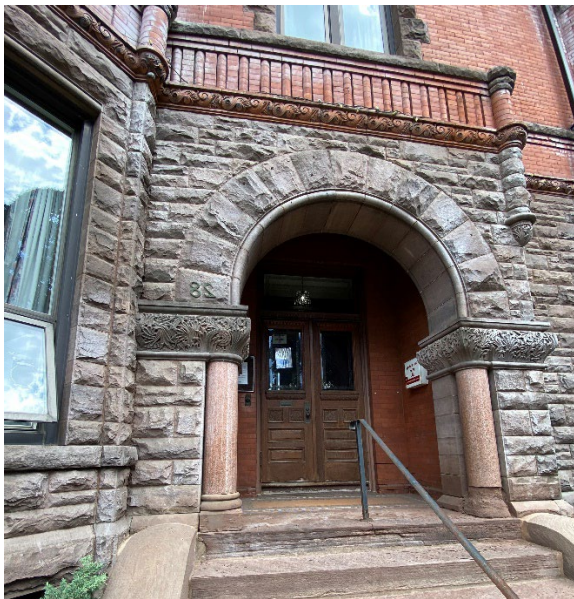
8. The front entrance with its segmental masonry and granite columns. Use of a variety of materials such as terracotta, stone, and brick provide visual interest and texture, characteristic of the Queen Anne Revival style. (Heritage Planning, 2024)
