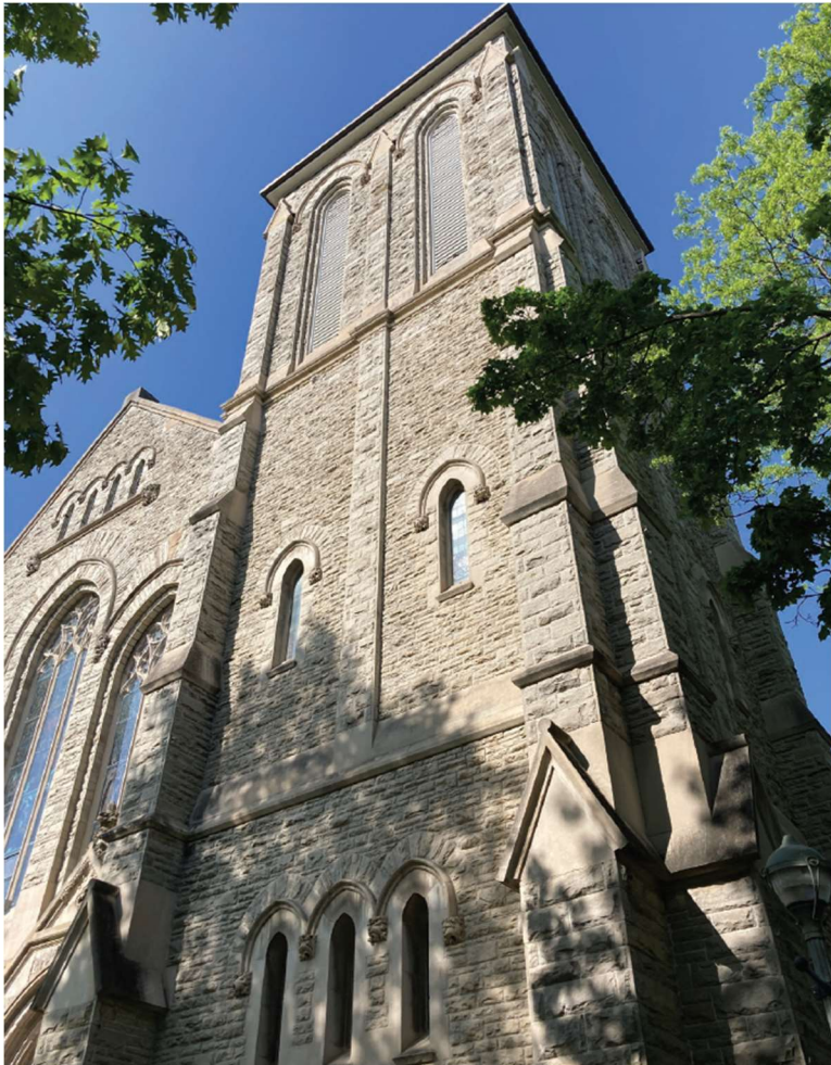
Figure 4 Detail of square tower with corner buttresses, lancet windows, and belfry with paired pointed arch openings (Heritage Planning, 2024).
