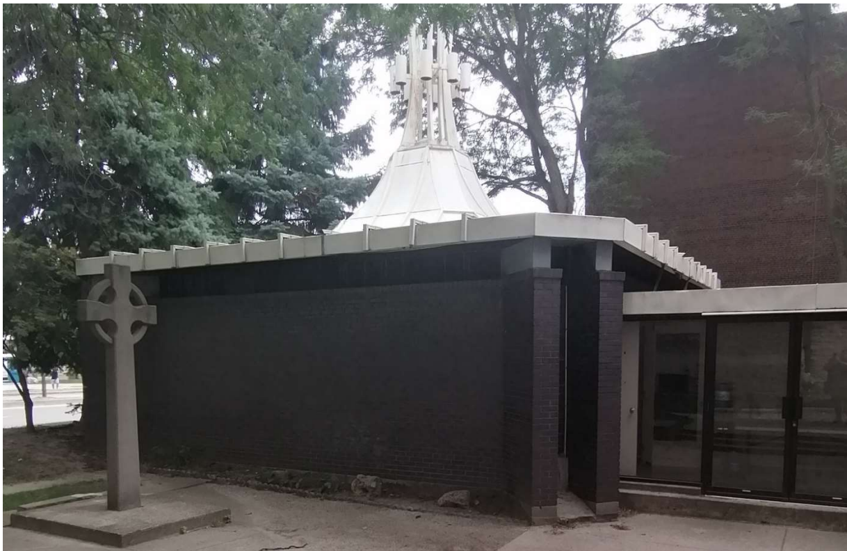
Figure 28 Southeast view of Chapel featuring corner buttresses, dark brick cladding and curved metal roof with finial of steel beams and cylindrical light fixtures. The Celtic Cross installed in 1961 is in the foreground (Heritage Planning, 2024).
