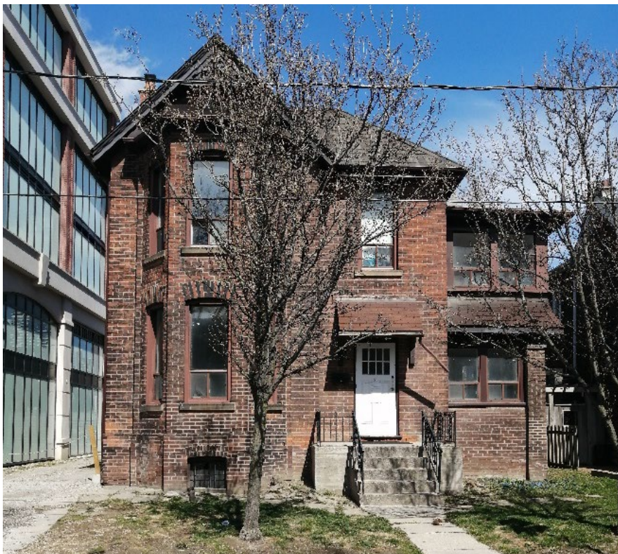
South elevation at 26 Millwood Road (Heritage Planning, April 2024).
