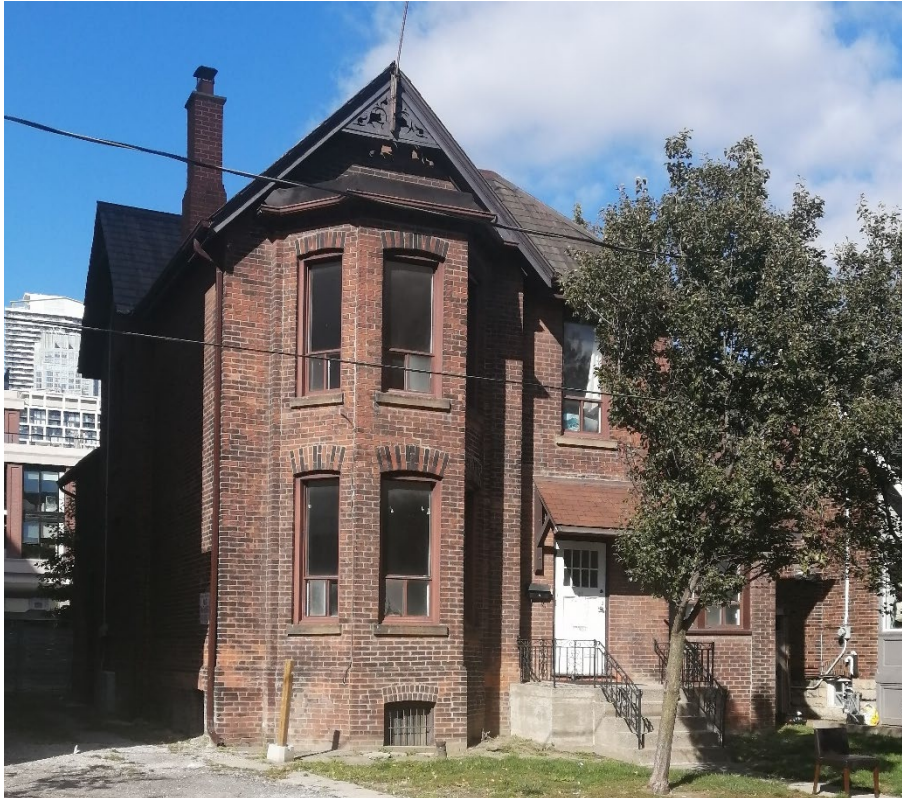
View of south and west elevations at 26 Millwood Road showing two-storey three-sided bay, brick voussoirs, stone sills and decorative gable pediments (Heritage Planning, October 2024).
