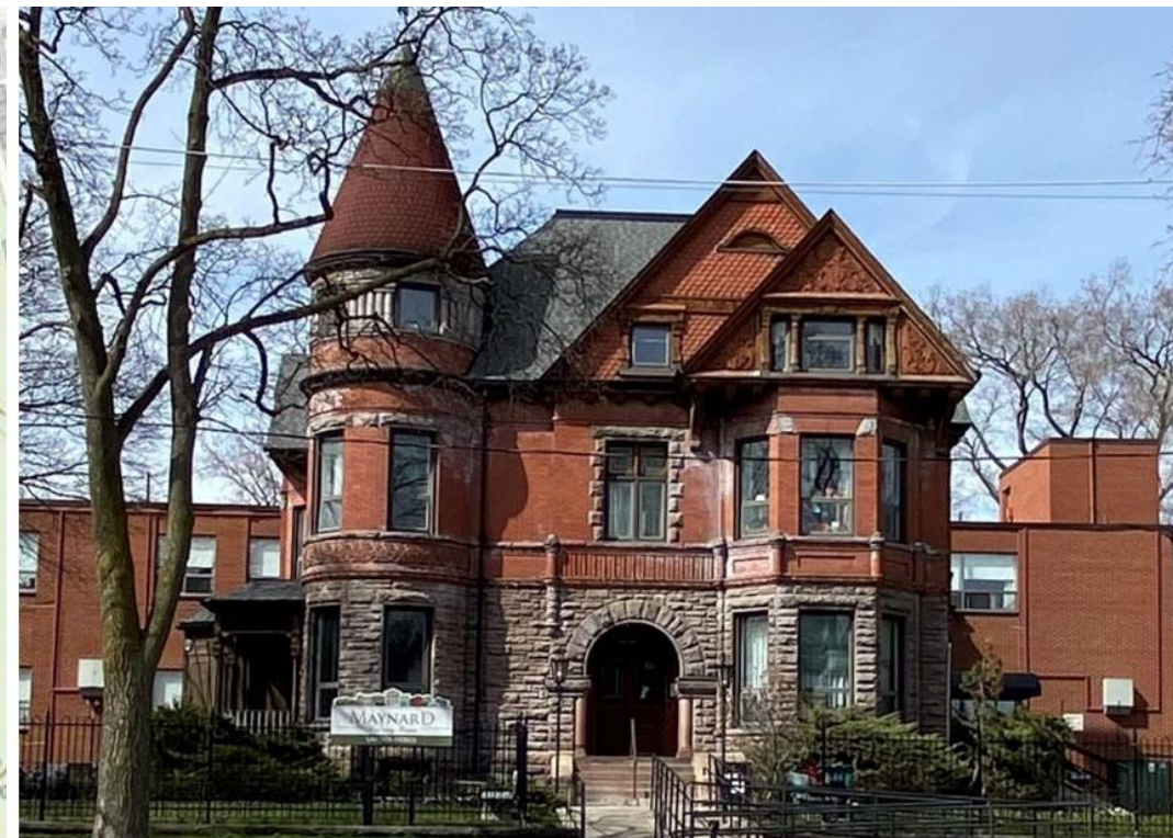
South elevation (principal) of 28 Halton Street (Heritage Planning, 2024)
