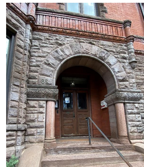
Recessed entrance and arched entryway in rusticated Credit Valley stone (bottom left) (Heritage Planning, 2024)
