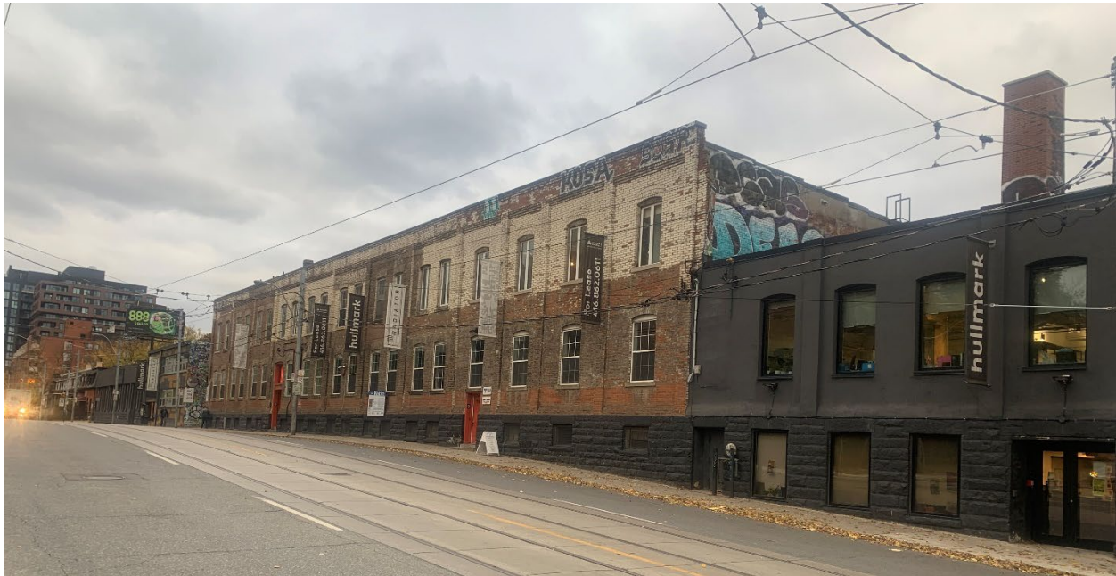
Image 28: Current photograph of 360 Dufferin Street, east elevation looking south with the remnant structure of 366-370 Dufferin Street adjoining at right. (Heritage Planning, 2024)
