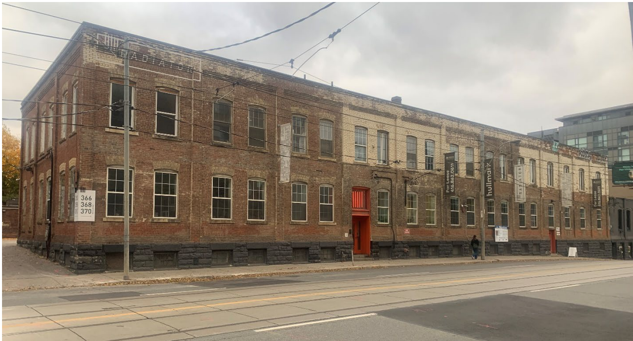
Image 27: Current photograph of 360 Dufferin Street, east and south elevations. Built in two phases, each of the 4 bays at right contain a single window at each storey while the later 8 bays contain pairs. (Heritage planning, 2024)
