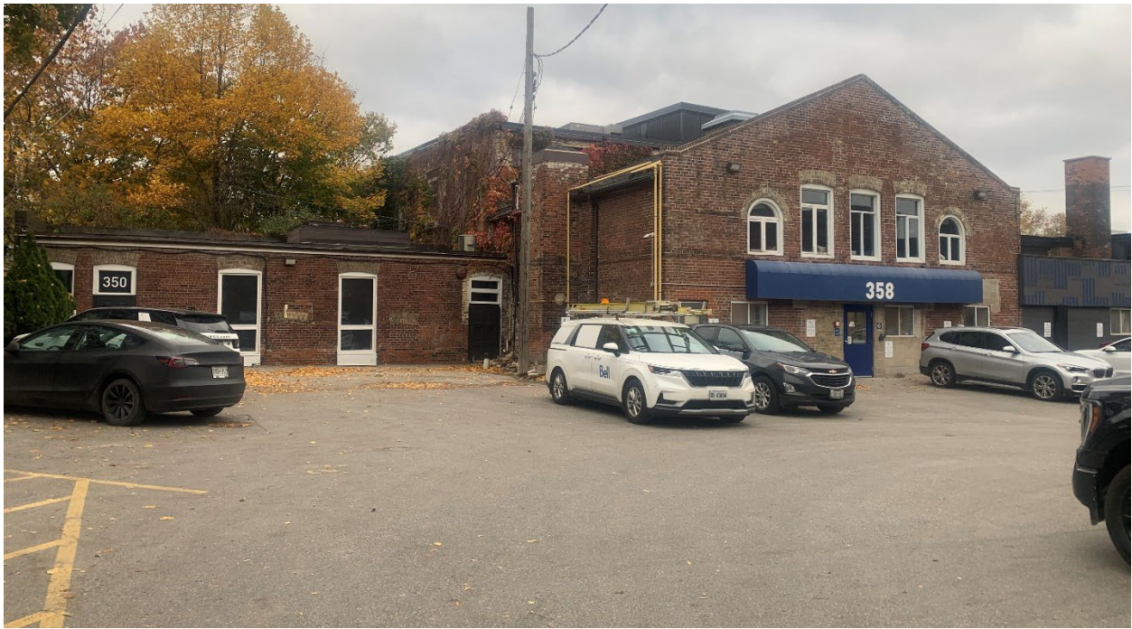
Image 20: Current photograph looking west at the Mixing building (350 Dufferin) and Core Oven building (358 Dufferin) from the central courtyard (Heritage Planning, 2024)
