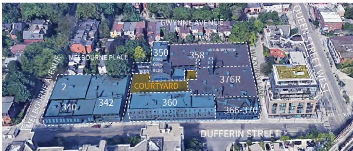
Aerial View of the Dominion Radiator Complex (Google Maps, annotated by ERA)
