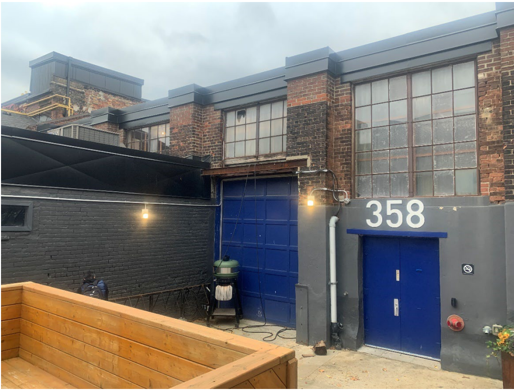
Image 25: Current photograph of the Foundry, east elevation (Heritage Planning, 2024)
