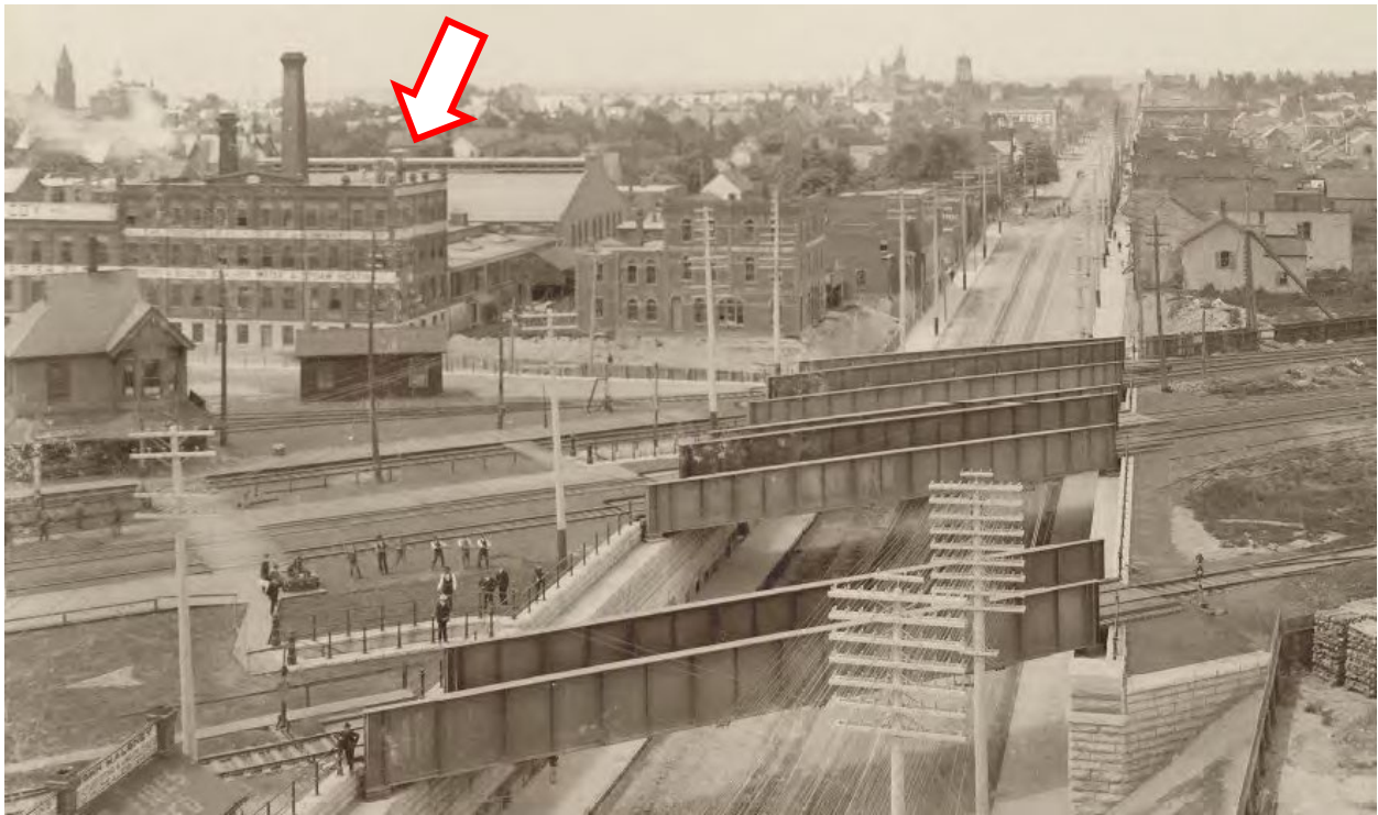
Image 6: c.1898 archival photograph looking west along Queen Street to Dufferin Street and the new rail overpass. The Dominion Radiator complex is indicated by the arrow. Note the full three storey plus exposed basement height of the building at 366-370 Dufferin Street and the gable roof with clerestory windows on the Foundry.
