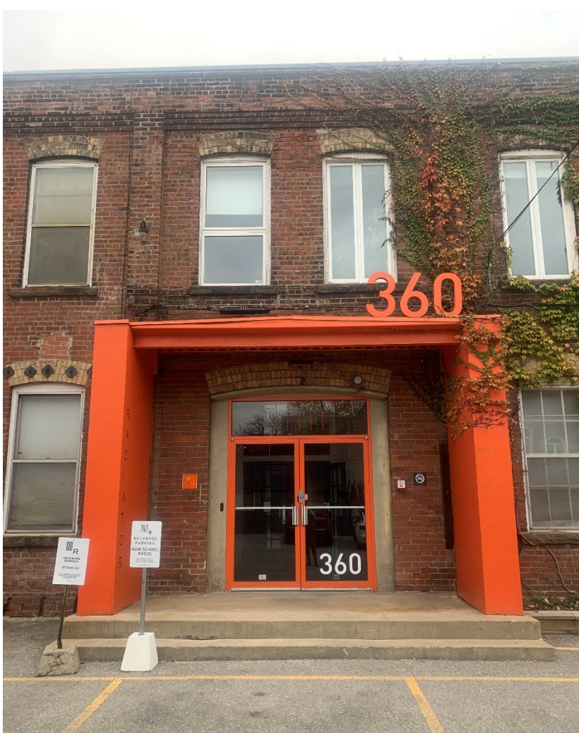
Image 32: 360 Dufferin Street, west elevation showing the main entrance onto the central courtyard. (Heritage Planning, 2024)
