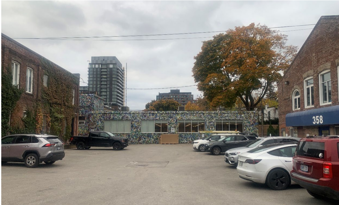
Image 18: Current photograph of the complex looking south from the central courtyard. (Heritage Planning, 2024)
