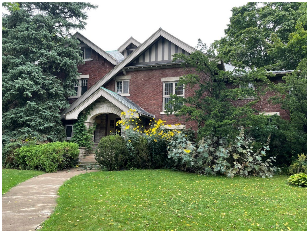
Main (west) façade of 94 Cortleigh Boulevard, 2024 (City of Toronto Heritage Planning)
