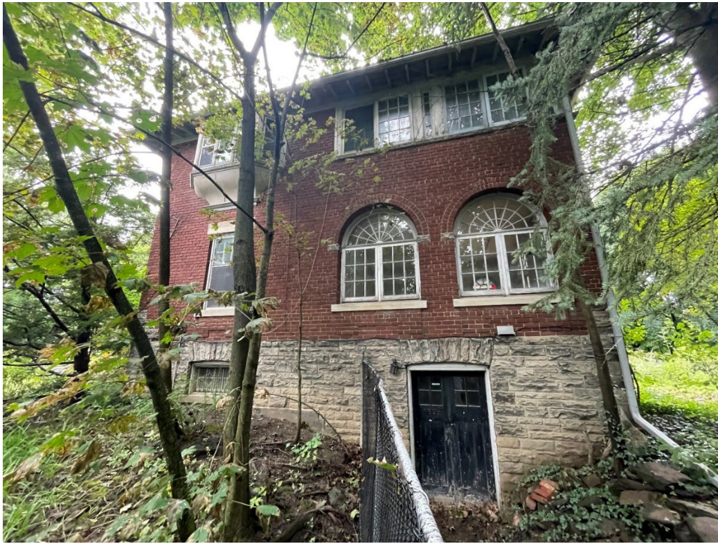
Figure 5: side (south) façade - note the cantilevered Jacobethan window on left side of second storey - 2024 (City of Toronto Heritage Planning)
