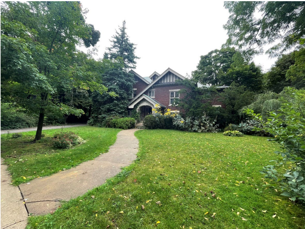
Figure 2: main (west) façade, 2024 (City of Toronto Heritage Planning)
