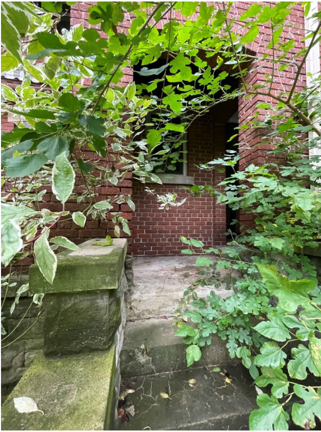
Figure 15: portion of rear façade (obscured by foliage) showing open, integral porch with stone stair wing walls, 2024 (City of Toronto Heritage Planning)
