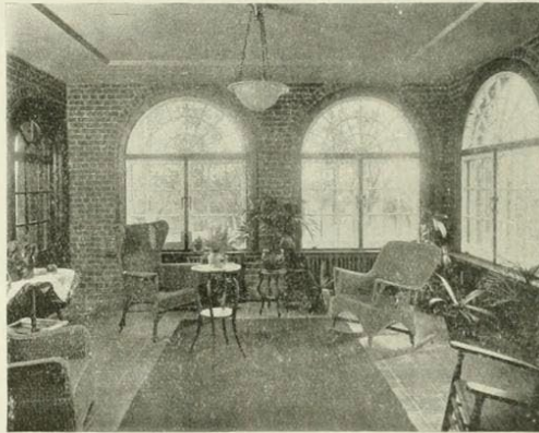
Fig. 11—Palm room on ground floor. Note flat bowl semi-indirect lighting fixture. Hardware supplied by Aikenhead Hardware, Limited.
