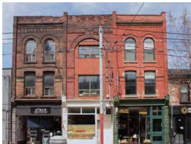
Figure 38: 1084-1086 1/2 Queen Street West are representative examples of the Italianate architectural style.
