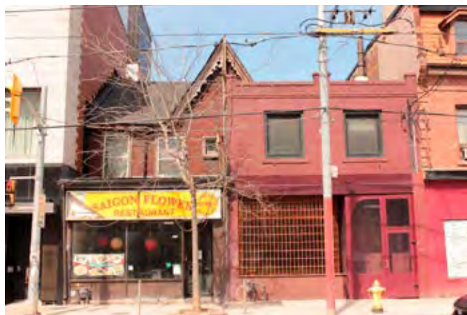
Figure 30: 1136-1138 Queen Street West are the only properties in the West Queen West HCD classified as examples of the House-form with Storefront Addition typology.
