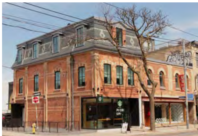
Figure 64: The same properties photographed in 2024, where the façade of 1026 Queen Street West has been restored and the polychromatic brick cladding of 1030 Queen Street West has been revealed.
