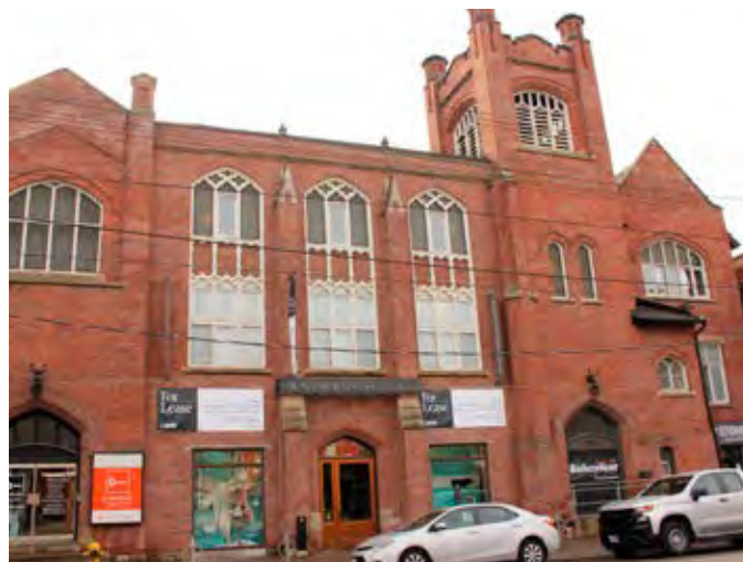
Figure 37: The former Euclid Avenue Methodist Church at 765 Queen Street West is a representative example of the Gothic Revival architectural style.
