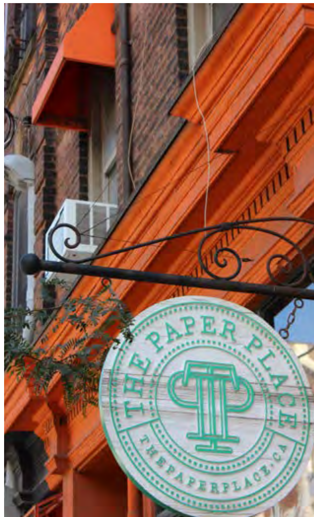
Figure 84: Example of a projecting sign mounted on the lower storey of the contributing property at 887 Queen Street West.
