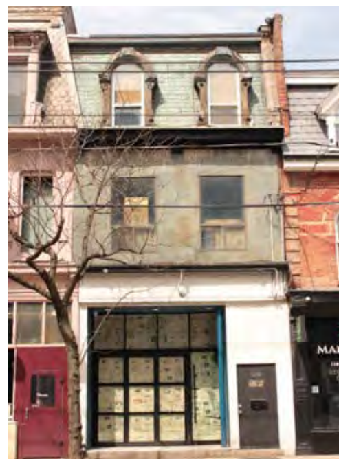
Figure 69: An over-clad building at 1166 Queen Street West whose historic building features may be restored with careful removal of the over-cladding.
