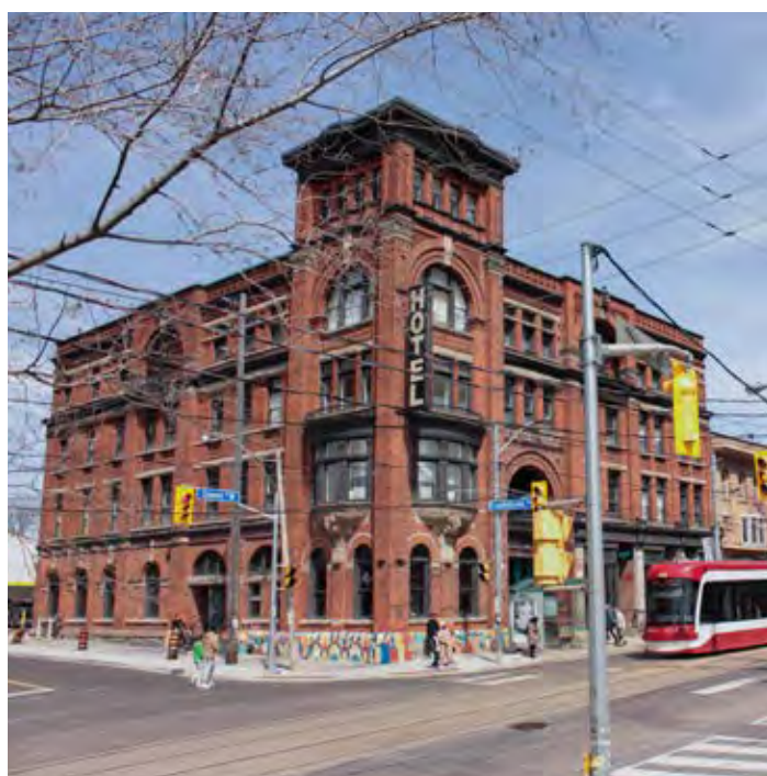
Figure 42: View 3, northeast towards the Gladstone Hotel at 1204 Queen Street West and Sudbury Street.
