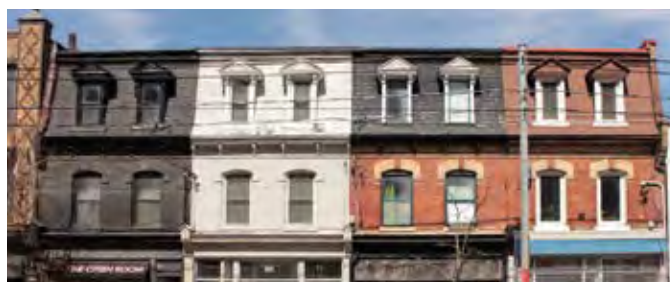
Figure 71: 974-982 Queen Street West are representative examples of properties with a mansard roof.
