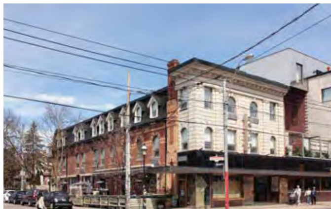
Figure 120: 1150 Queen Street West photographed in 2024, after the restoration and revitalization work that took place in the 2000s.
