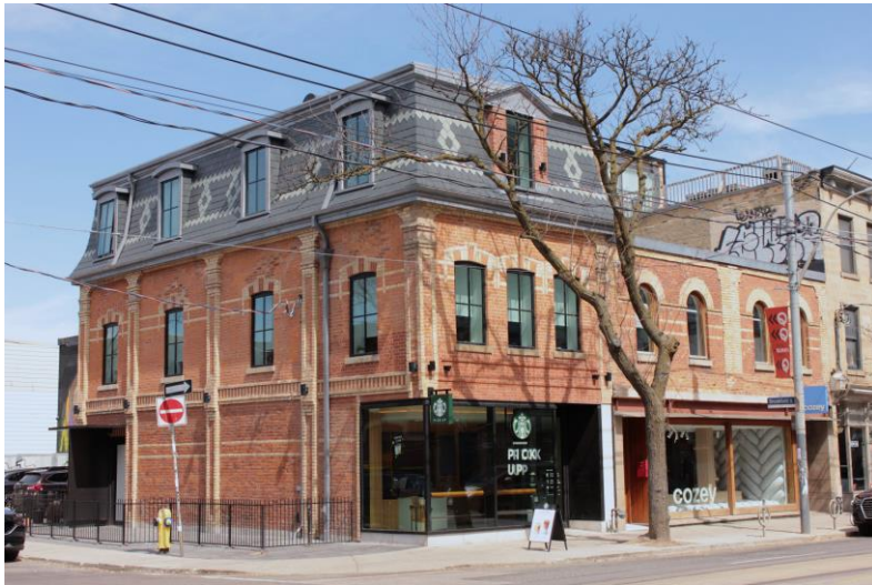
CONTRIBUTING PROPERTIES 1026 and 1030 Queen St W
