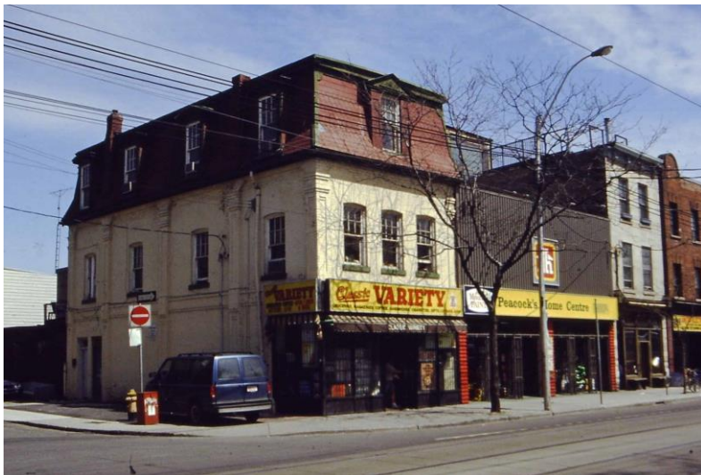
CONTRIBUTING PROPERTIES 1026 and 1030 Queen St W photographed in 1992 (CTA)
