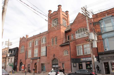
Former Euclid Avenue Methodist Church at 765 Queen St W
