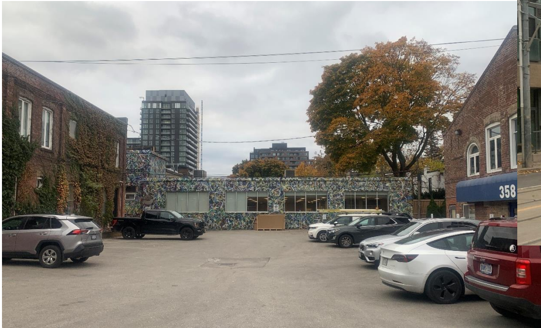
Above: Looking south across the central courtyard with the Factory Offices at left and the Core Oven Building at right
