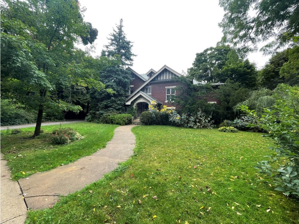
above: main (west) façade, 2024 (City of Toronto Heritage Planning)
