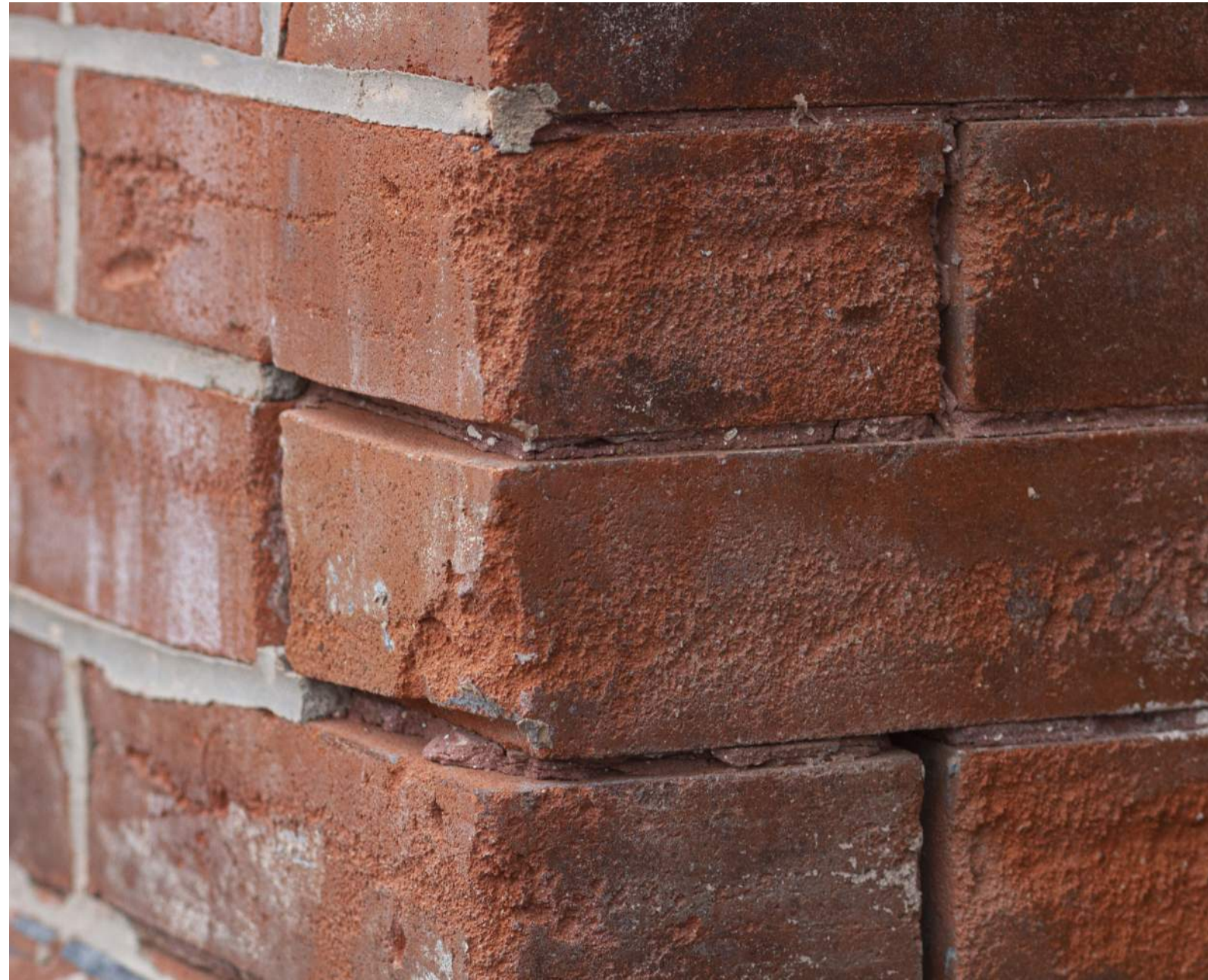
Contrast between former fine mortar joints (right) and saw-cut joints
