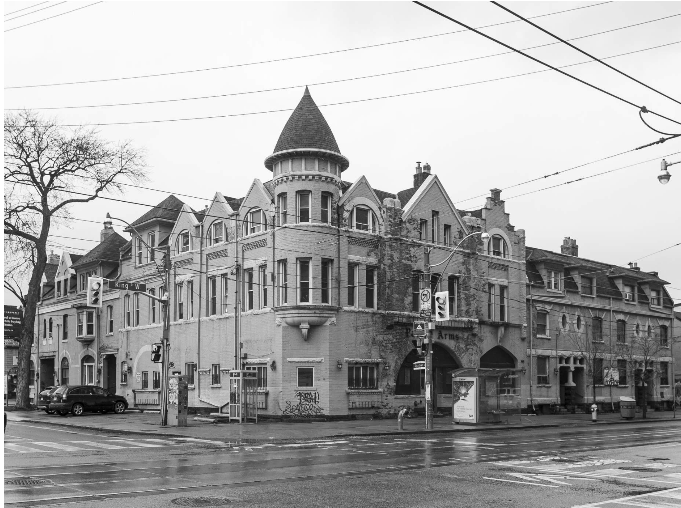
View looking towards the southwest corner of the building, Photographer: Dan Chan, 2022
