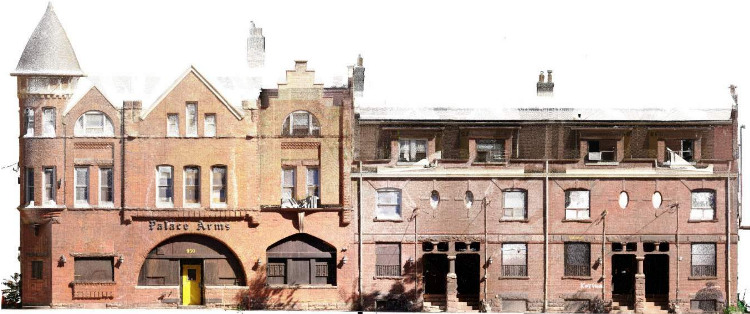
3D LiDAR scan of existing building, South Facade, captured 2023
