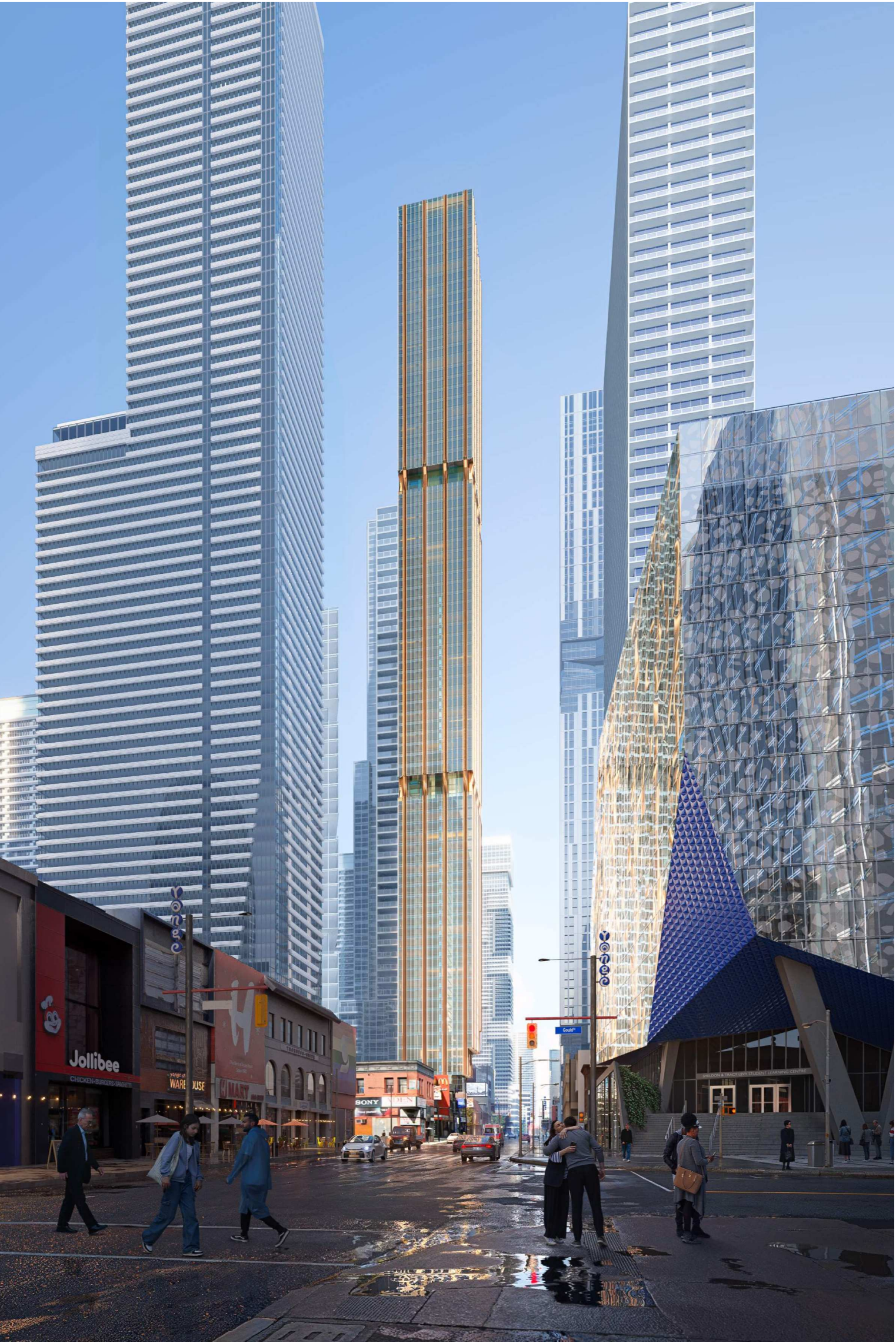
View from the South
