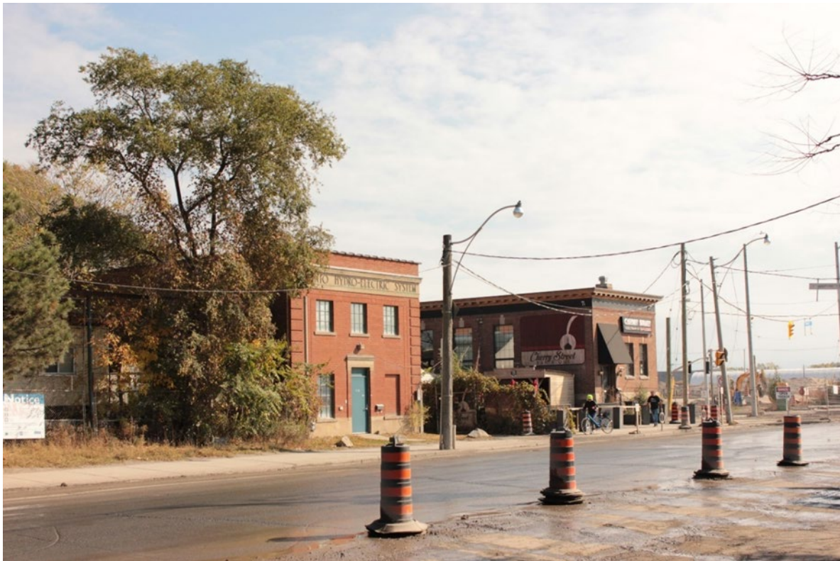
Figure 40. Toronto Hydro Station and former Dominion Bank at the corner of Cherry and Commissioners streets (Heritage Planning, 2023).
