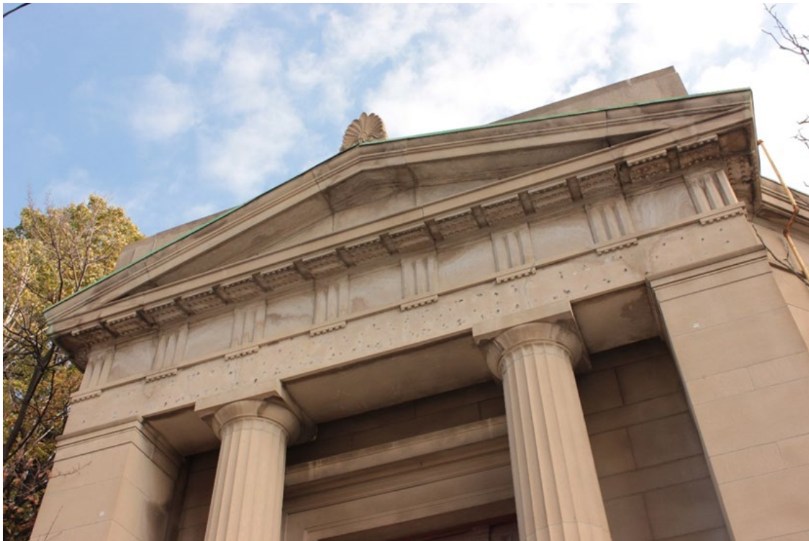
Figure 15. Pediment and entablature detail (Heritage Planning, 2023).
