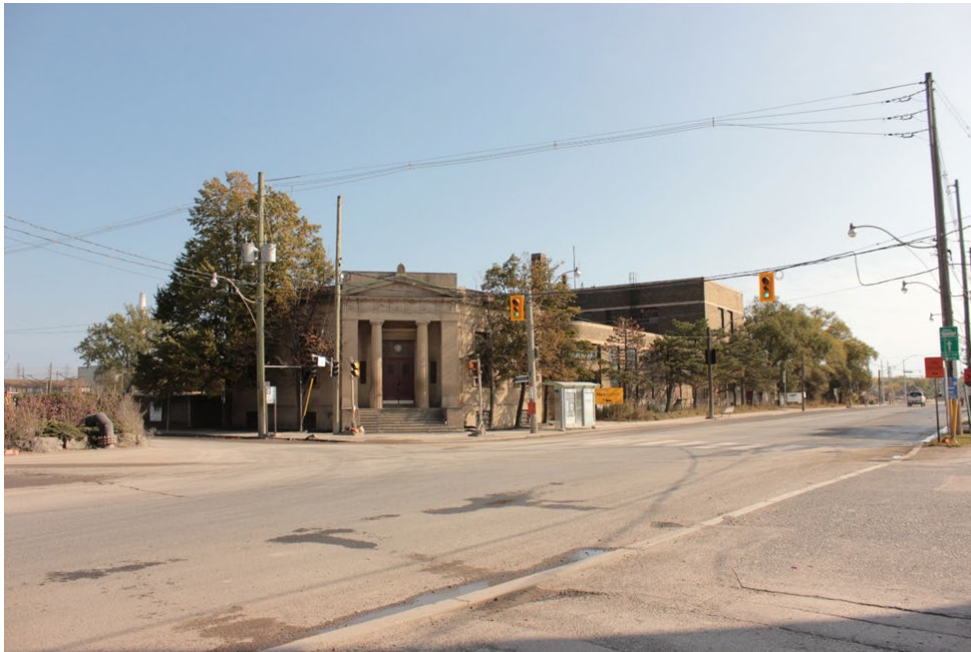
Figure 35. Intersection of Cherry and Villiers streets, facing southeast (Heritage Planning, 2023).
