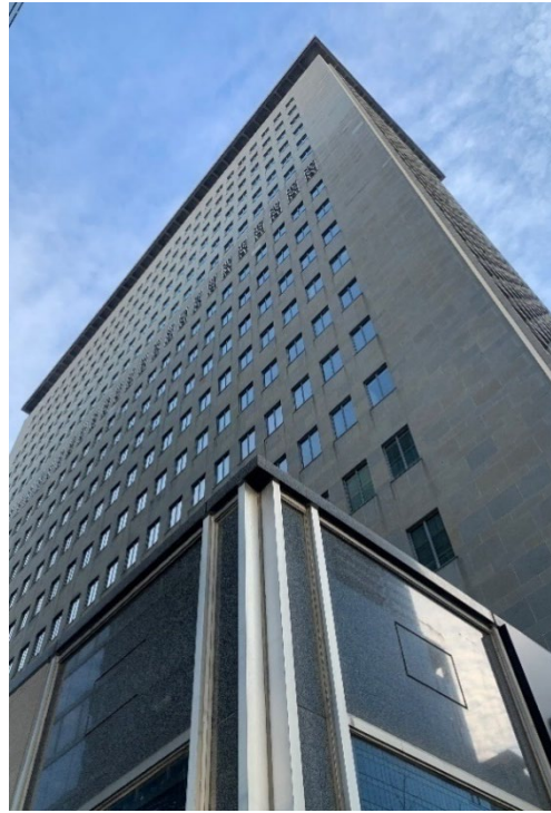
Images 31 and 32. At left, the west elevation showing the raised stone 'fins' rising vertically between the window bays; at right, the north elevation showing the metal 'fins' on the Norwegian Blue Granite podium. (Heritage Planning, 2023)
