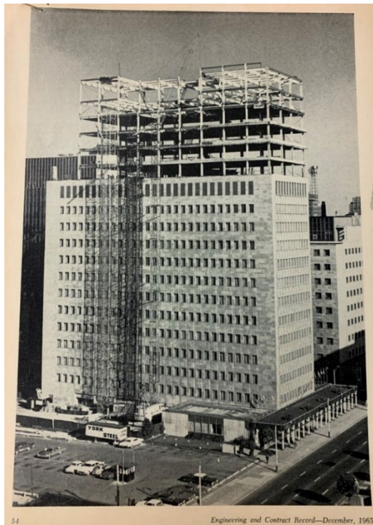
Images 17 and 18. 1965 article featuring the modified mobile tower crane used to hoist the structural steel necessary for the Shell Oil Building's 7-storey addition. (Engineering and Contract Record)
