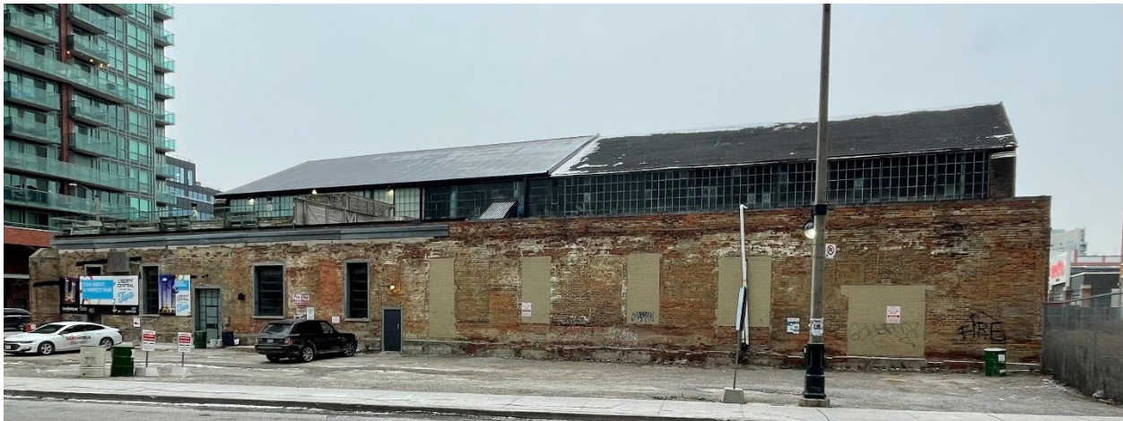
Figure 13. East elevation of the A. R. Williams Machinery Company Warehouse. The former prison building's interior (party) wall now forms the east exterior wall of the A. E. Williams Machinery Company Warehouse, 2024 (Heritage Planning)
