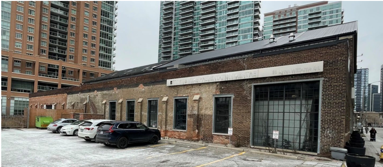
Figure 12. West elevation of the A. R. Williams Machinery Company Warehouse, 2024 (Heritage Planning)
