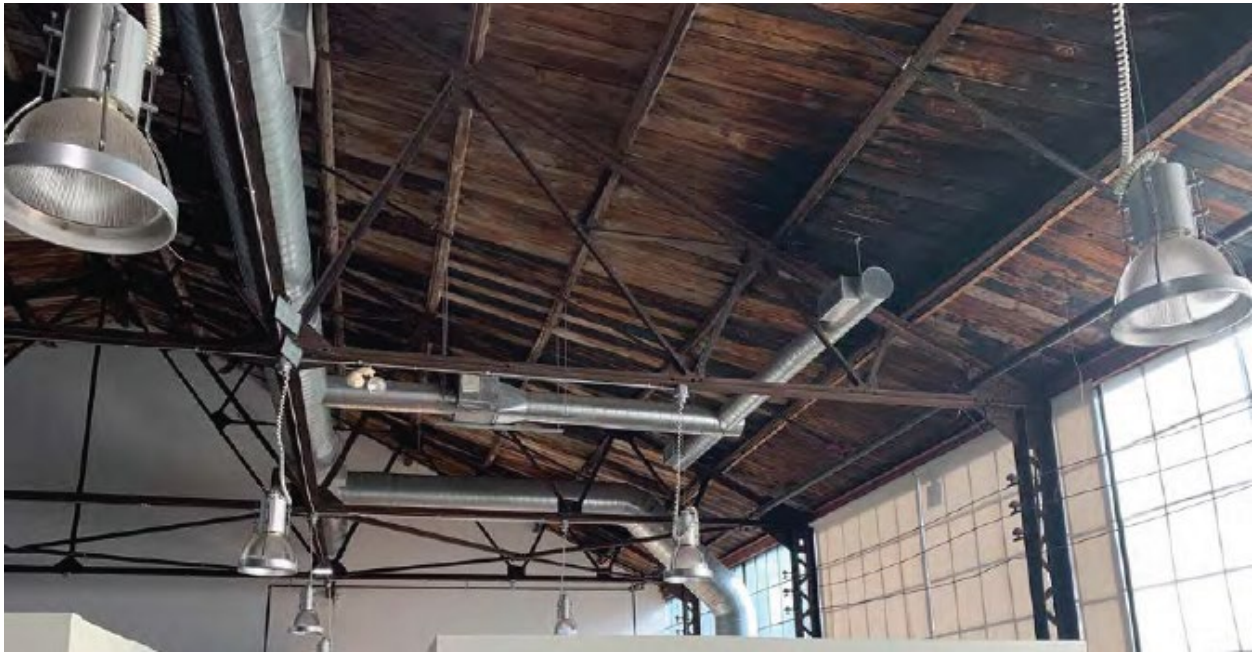
Figure 16. Interior view of the A. R. Williams Machinery Company Warehouse showing steel truss ceiling, 2023 (Heritage Impact Assessment, E.R.A. Architecture)
