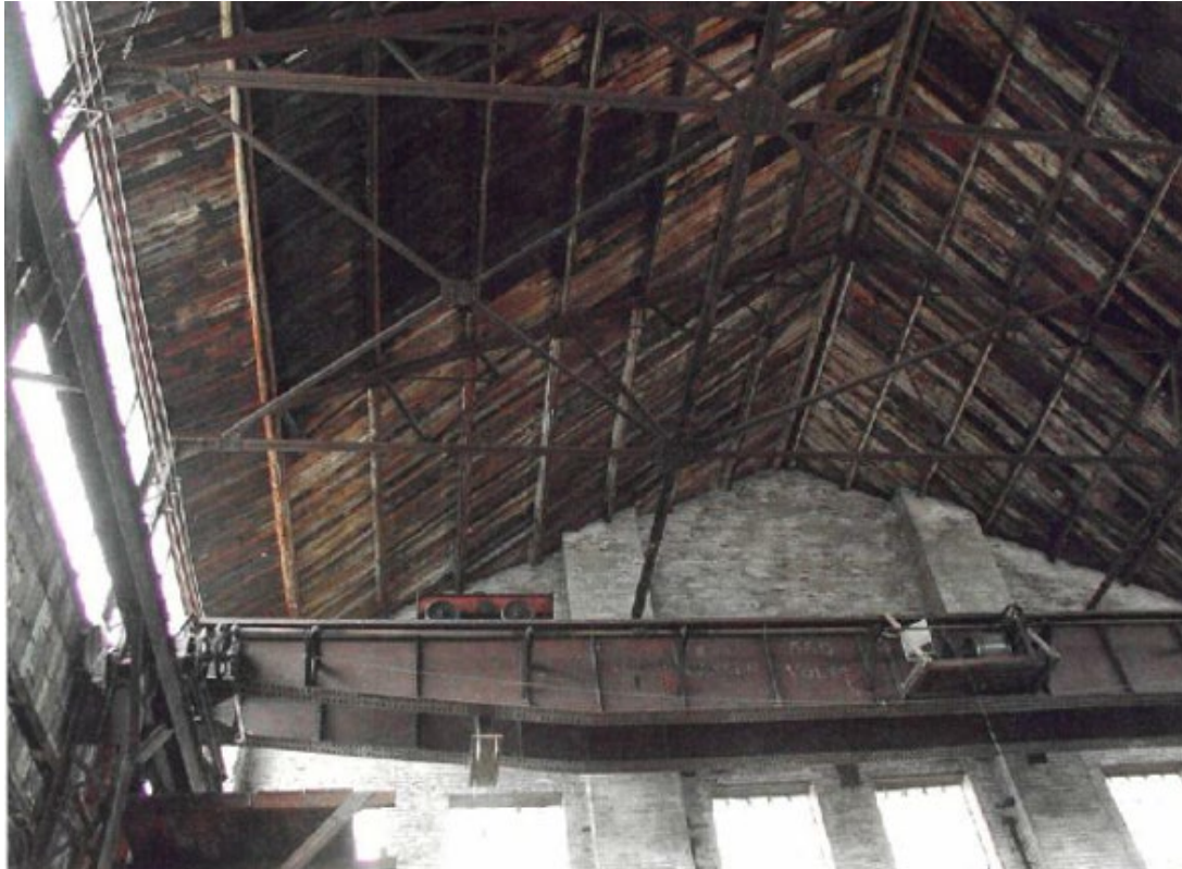
Figure 19. Interior view of the A. R. Williams Machinery Company Warehouse showing the travelling crane, c. 2005 (Heritage Planning)
