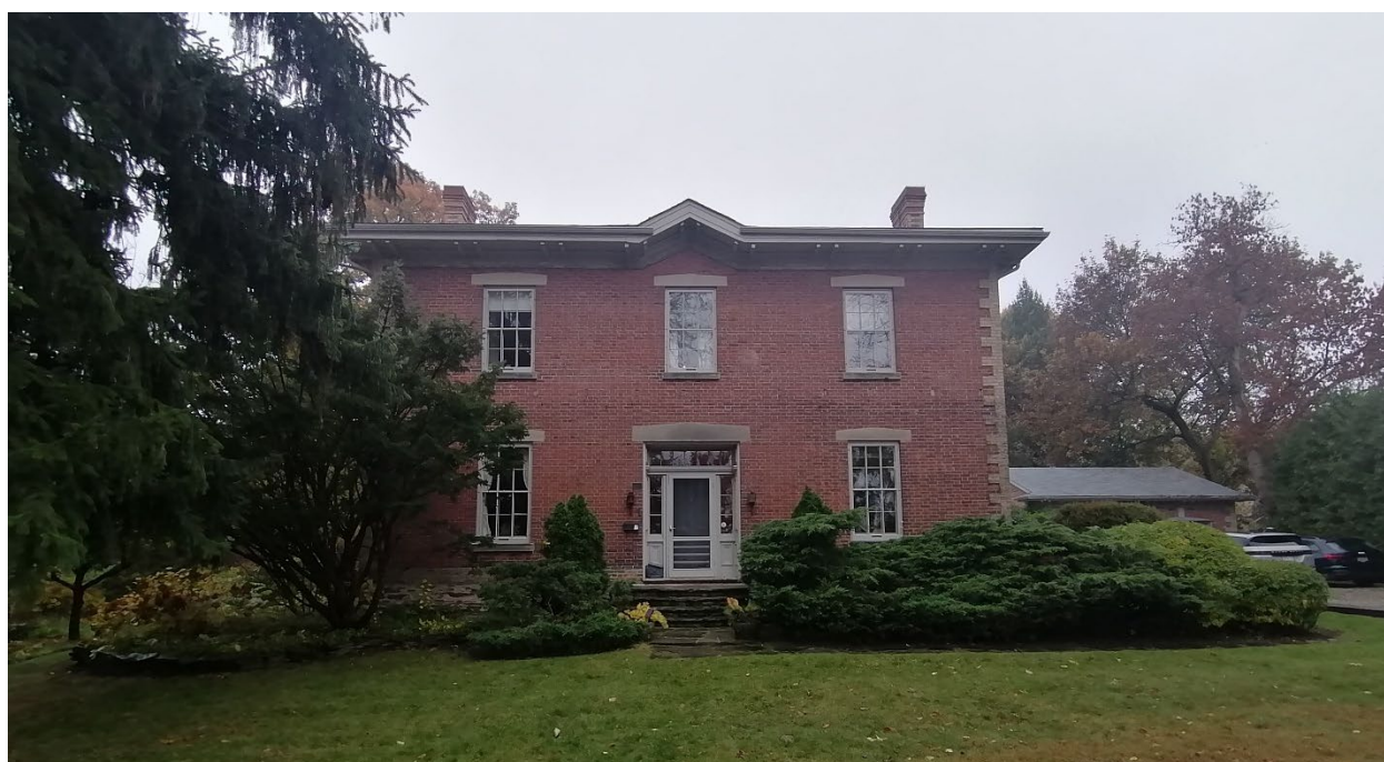
View of principal (east) elevation at 1 Heritage Place (Heritage Planning, 2023).
