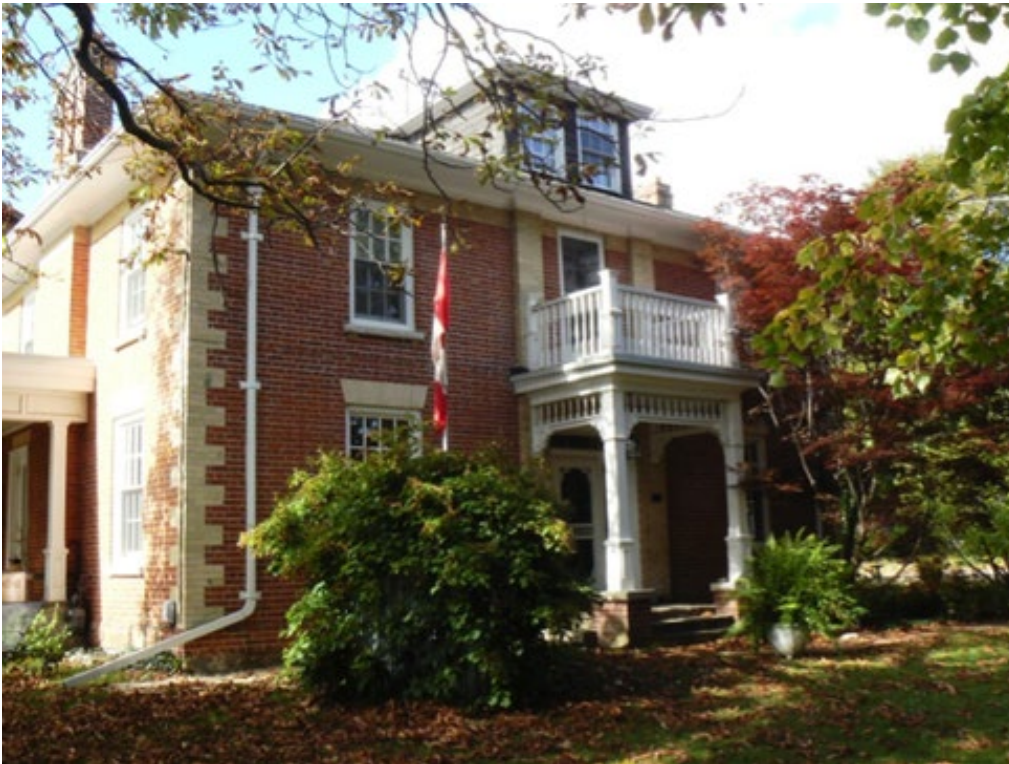
16. Image of the George W. Thompson House at 7 Meadowcrest Road (Listed). Designed and built between 1855 and 1860 by William Tyrrell, it shares many elements with 1 Heritage Place including square massing, hipped roof, fenestration, buff brick quoining, and deep eaves (Etobicoke Historical Society).
