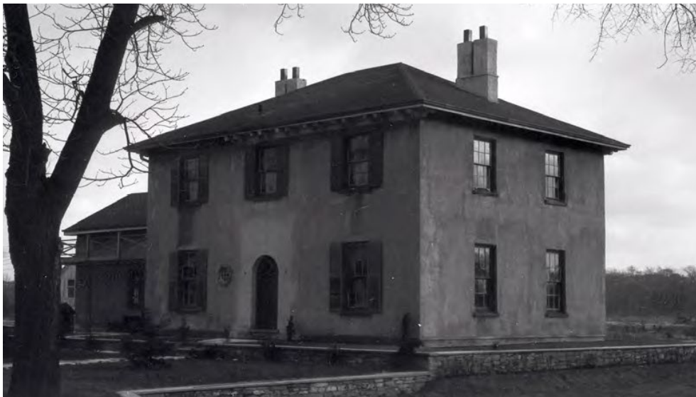
14. Image of the Dennis family's historic Buttonwood Estate (Demolished). Constructed on the east side of the Humber River in c.1852 by William Tyrrell it shares many elements with 1 Heritage Place including square massing, hipped roof, fenestration, and deep bracketed eaves (City of Toronto Archives).
