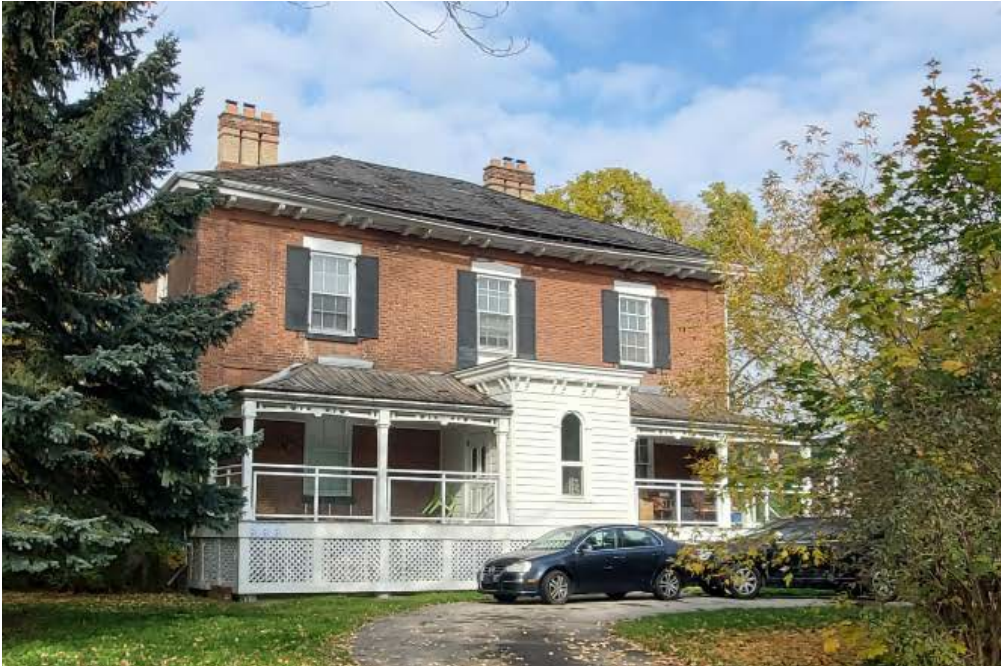
15. Image of the William Tyrrell House at 64 King Street in Weston (Designated). Designed and built c.1859 by William Tyrrell it shares many elements with 1 Heritage Place including square massing, hipped roof, fenestration, deep bracketed eaves, rear ell, and stone square and triangular stone lintels (Heritage Planning, 2021).
