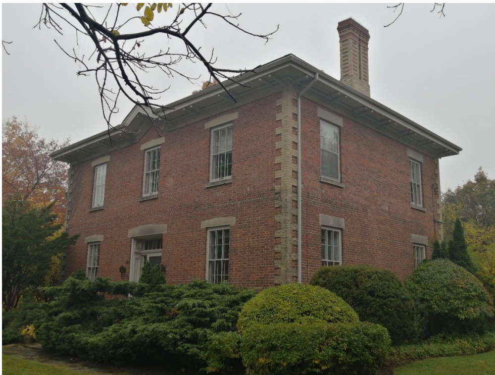
4. View of 1 Heritage Place looking south, showing the principal (east) and north elevations of the main structure with stone lintels and sills, buff brick quoining, six-over-six windows, chimney, and deep eaves with lambs tongue brackets (Heritage Planning, 2023).
