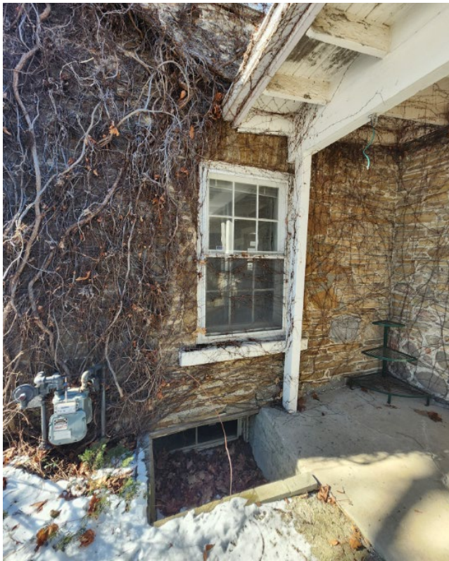
Figure 20. Detail of the rear (east) elevation of the main house illustrating the first storey window and Humberstone (Heritage Planning, 2024)
