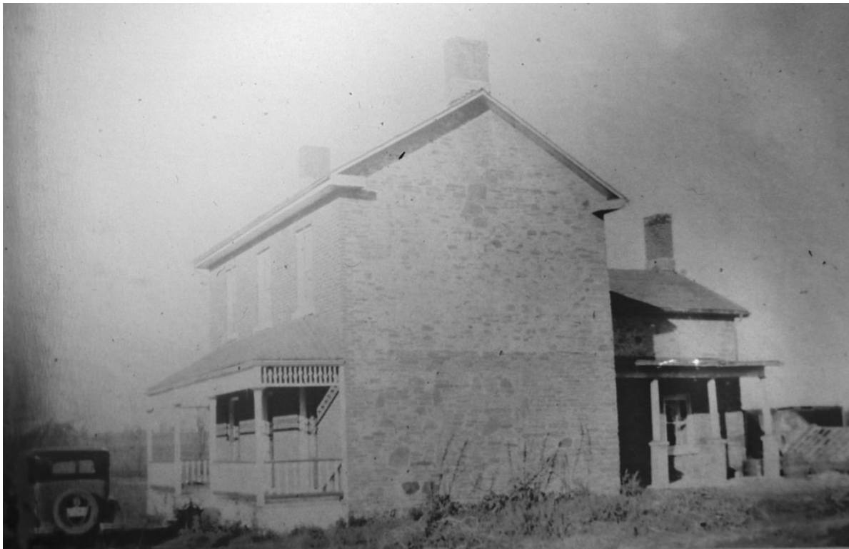
Figure 6. Historic photograph looking north at the main house (left) and rear kitchen wing (right) and 322 La Rose Avenue (Etobicoke Historical Society)
