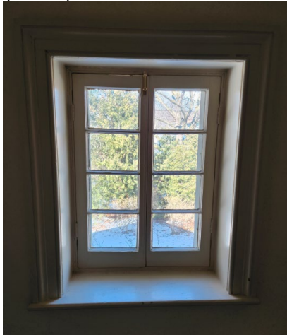
Figure 27. Detail of the casement of the window in the second storey of the side (north) wall of the rear kitchen wing (Heritage Planning, 2024)
