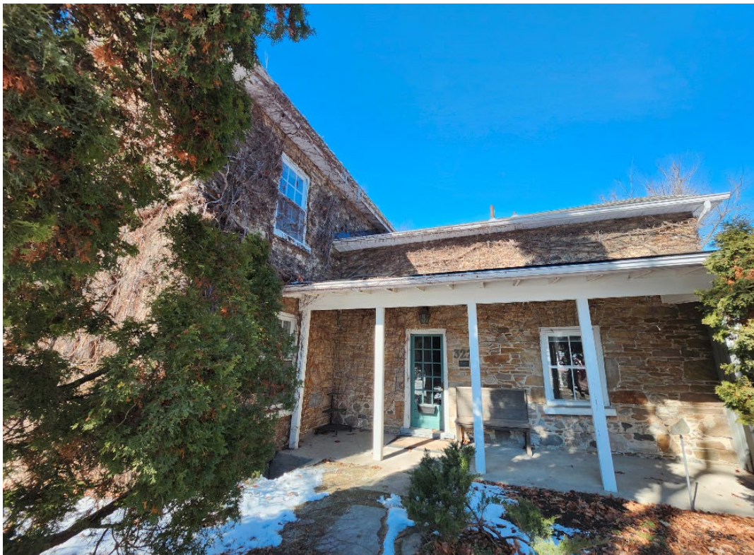
Figure 17. Detail of the current primary (south) elevation and main entryway to the property at 322 La Rose Avenue (Heritage Planning, 2024)
