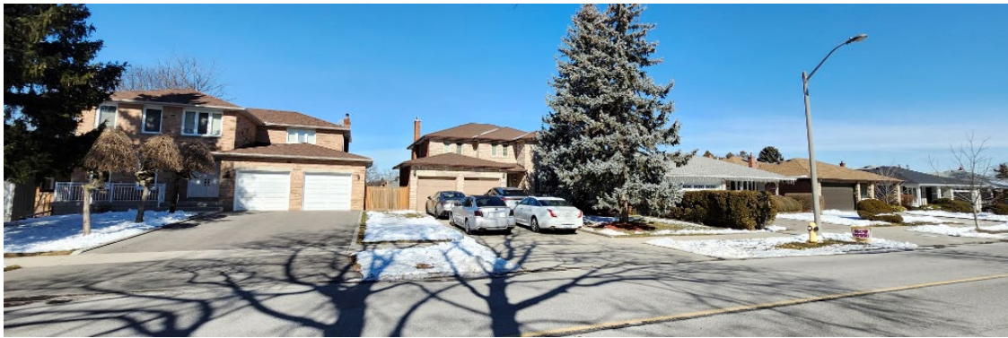
Figure 29. View looking at the north side of La Rose Avenue, east of the subject property, illustrating the post-1960s residential dwellings that populate the area (Heritage Planning, 2024)
