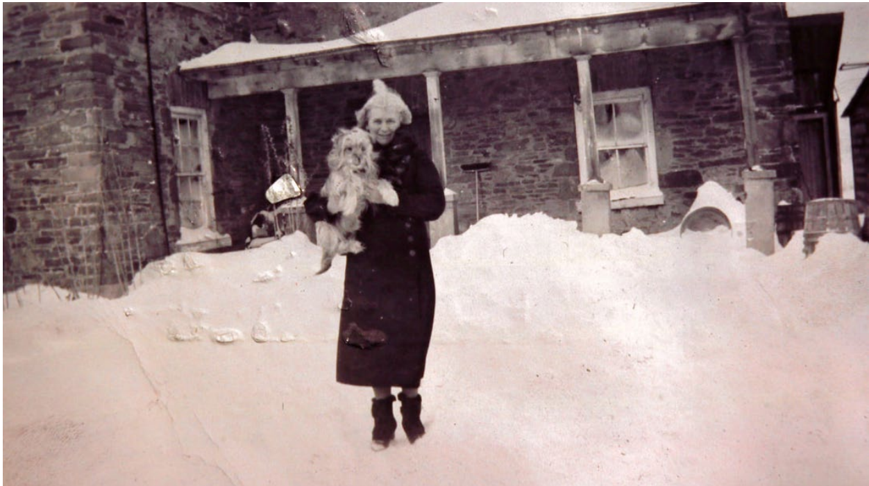
Figure 8. Historic photograph showing the rear kitchen wing and entrance (Etobicoke Historical Society)
