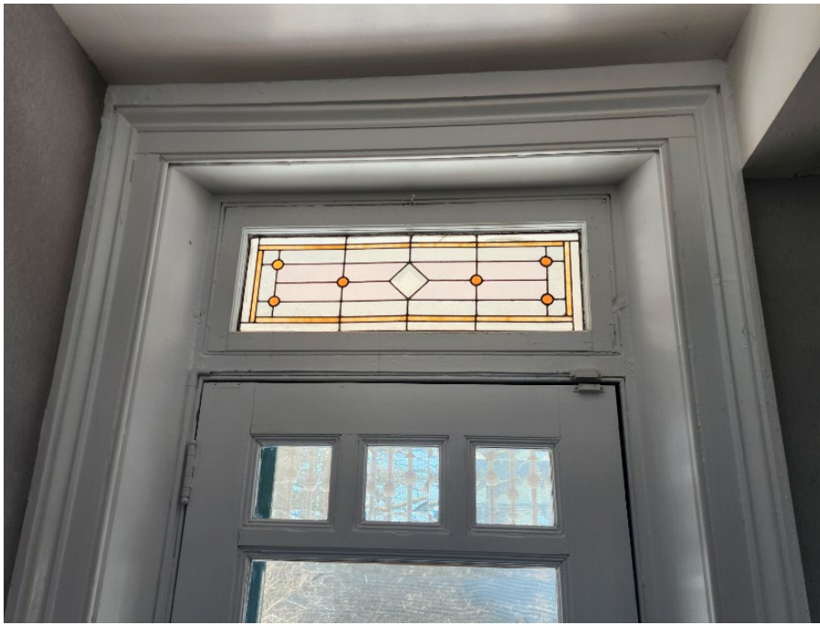
Figure 18. Detail of the transom above the door in the original primary (west) elevation of the main house (Heritage Planning, 2024)
