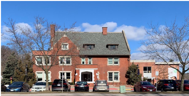
20. The estate house at 296 Lawrence Avenue East reflecting a more restrained application of Tudor Revival and Queen Anne Revival styles. Later additions built on the sloping table land (c.1960s and 2002) are visible to the right (Heritage Planning, 2024)
