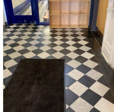
23. Detail of original black & white floor tiling (Heritage Planning, 2024)
