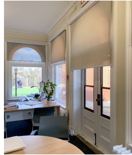
19. Details of the solarium with original wood double door and windows with an internal venting system along with an original cast iron radiator (Heritage Planning, 2024)
