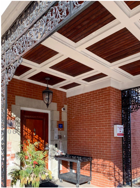
16. All three structures are unified by their centrally placed porte-cochère here in decorative metal with a beamed tongue and groove ceiling and original light fixture (Heritage Planning, 2024)
