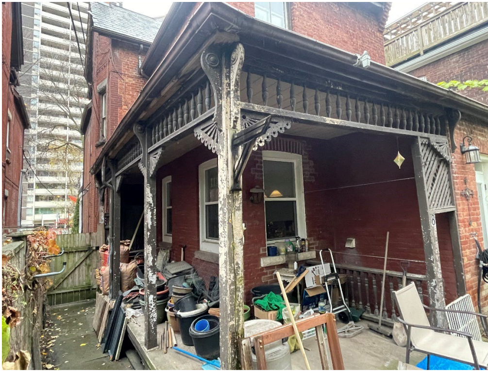
Figure 24: 8 Cawthra Square, rear verandah with spindle work detailing, 2023 (City of Toronto Heritage Planning)
