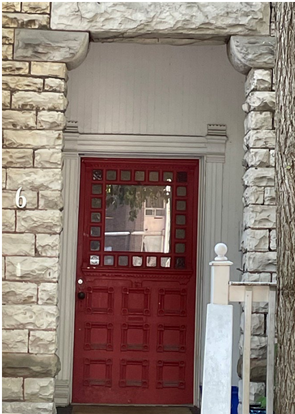
Figure 18: 6 Cawthra Square recessed entry showing Queen Anne-style wood panelled door, doorway casings and wooden tongue-and-groove wall cladding, 2023 (City of Toronto Heritage Planning)
