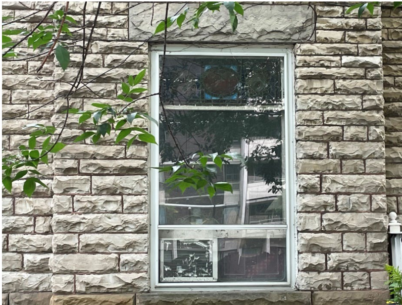
Figure 17: 6 Cawthra Square, detail view showing an example of the window sashes with leaded and stained glass transom light (behind modern storm sash), 2023 (City of Toronto Heritage Planning)
