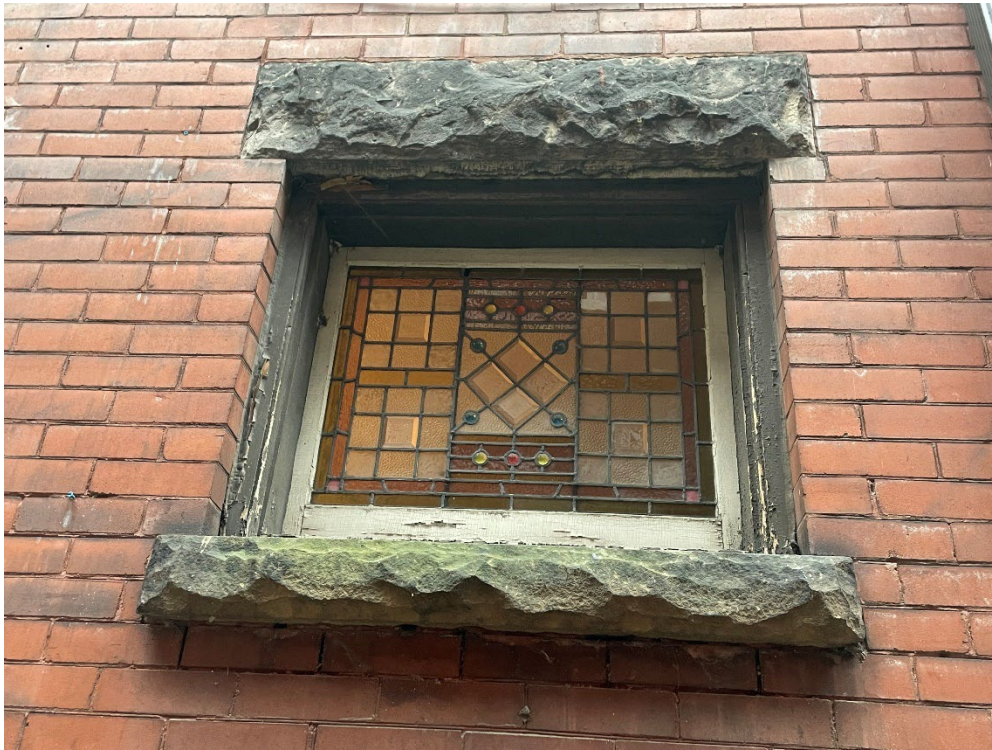
Figure 26: 8 Cawthra Square, east facade stained and leaded glass window, 2023 (City of Toronto Heritage Planning)
