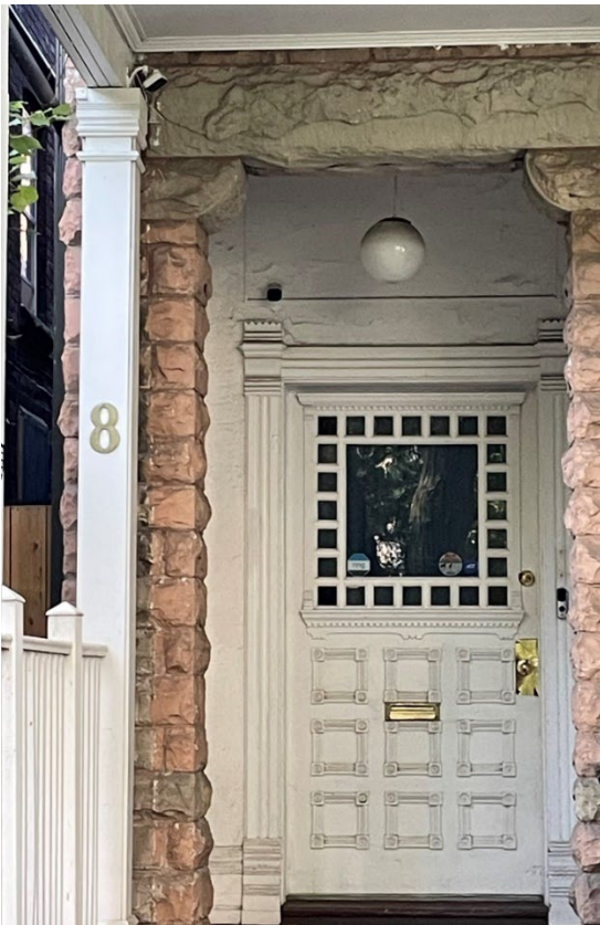
Figure 27: 8 Cawthra Square recessed entry showing Queen Anne-style wood panelled door, and doorway casings, 2023 (City of Toronto Heritage Planning)
