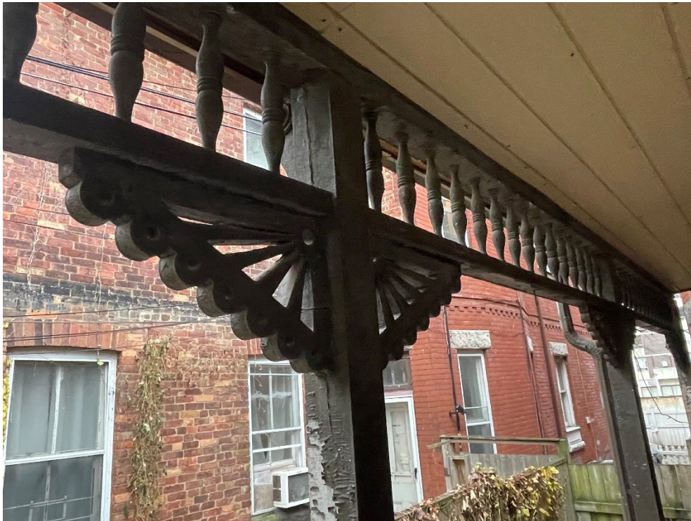
Figure 25: 8 Cawthra Square, detail view of rear verandah spindle work detail, 2023 (City of Toronto Heritage Planning)
