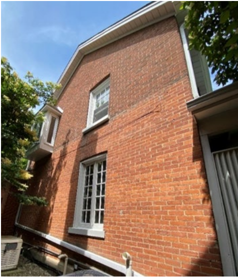
11. Partial view of the south elevation showing the ghost line of the former verandah, the two original flat or jack arch voussoirs, and the non-original bay window. The former south elevation entrance, beneath the bay window, has been bricked over (Heritage Planning, 2023).
