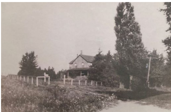
4. Partial view of the south elevation of 24 Mason Blvd. in 1915 showing the original verandah and part of the rear wing addition to the left of the building. Note that the rear wing once had a chimney; this was removed in 1999 (Ted Chirnside, North York Historical Society).
