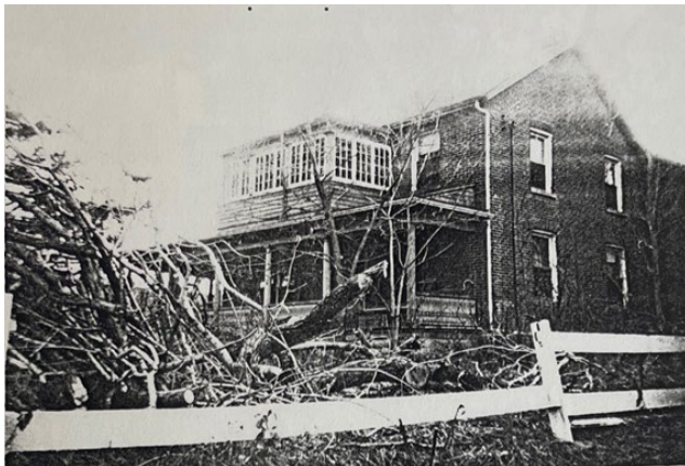
6. View of the east and north elevations of 24 Mason Blvd showing the original verandah, the sleeping porch, and the original configuration of the windows on the north elevation (North York Historical Society, 1966, NYCL).
