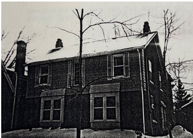
7. View of the front (east) elevation of 24 Mason Blvd. The verandah and sleeping porch have been removed. Note the awning added to the bottom right opening on the north elevation, indicating the new entrance (North York Historical Society, 1971, NYCL).
