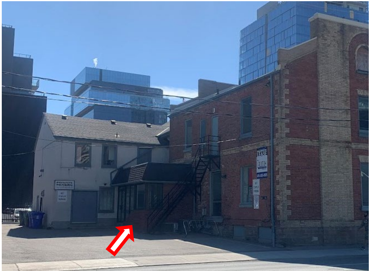
Figure 17. Current photo showing the single-storey enclosed rear entrance accessible to both the north elevation of the rear wing at 111, at left, and to the east elevation at 115 Berkeley, at right (Heritage Planning, 2024)
