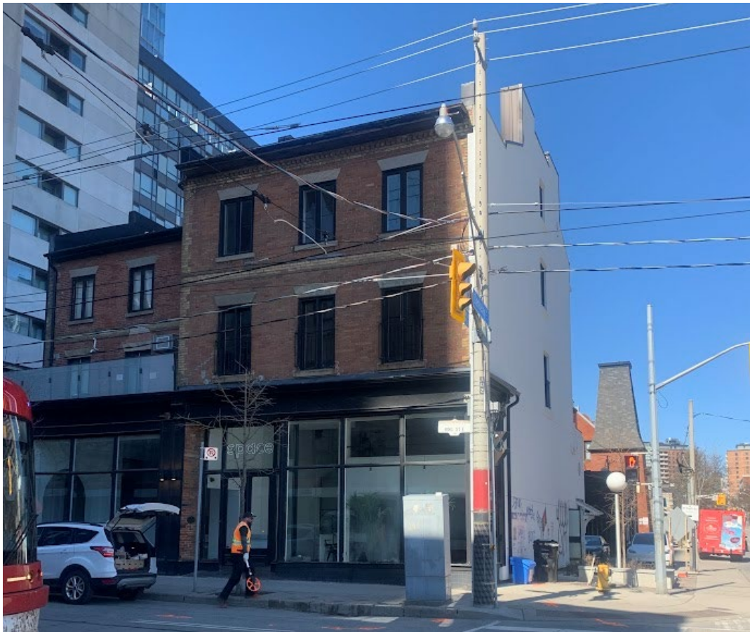
Figure 18. South elevation of the 1845 Charles Coxwell Small House located at the northwest corner of Berkeley and King Street East (Heritage Planning, 2024)
