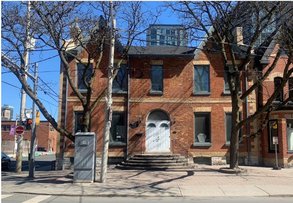
Figure 9. West elevation of 115 Berkeley Street (Heritage Planning, 2024)
