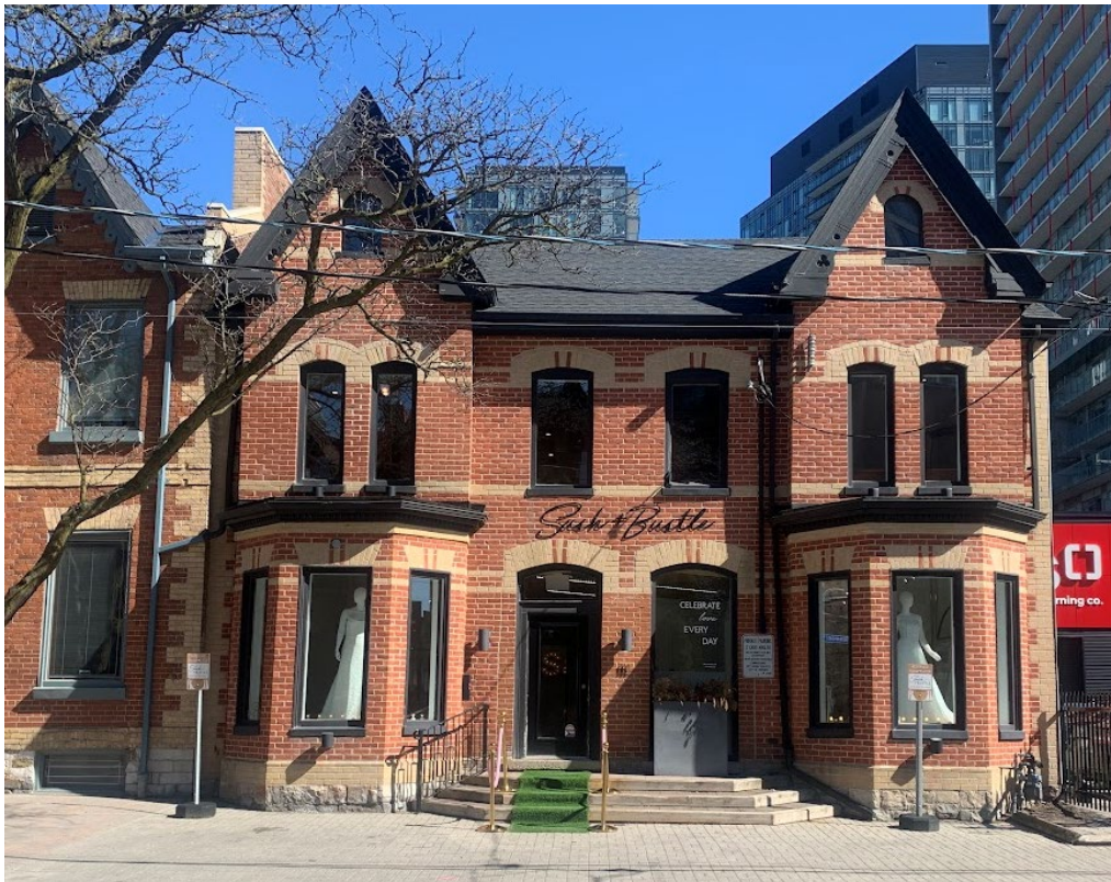
Figure 4. West elevation of 111 Berkeley Street (Heritage Planning, 2024)
