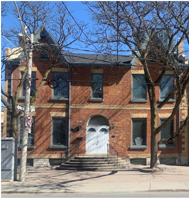
115 Berkeley Street (Heritage Planning, 2024)
