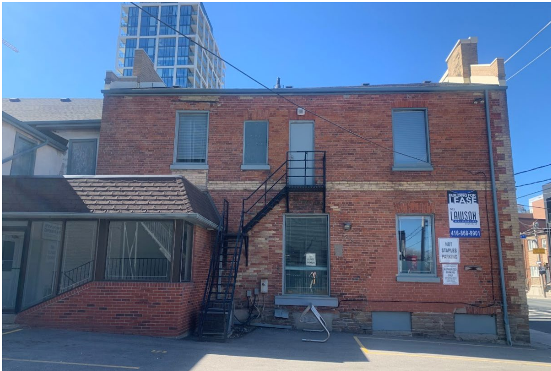
Figure 12. Rear (east) elevation at 115 Berkeley Street with later fire escape and one-storey enclosed stair entrance at left (Heritage Planning, 2024)
