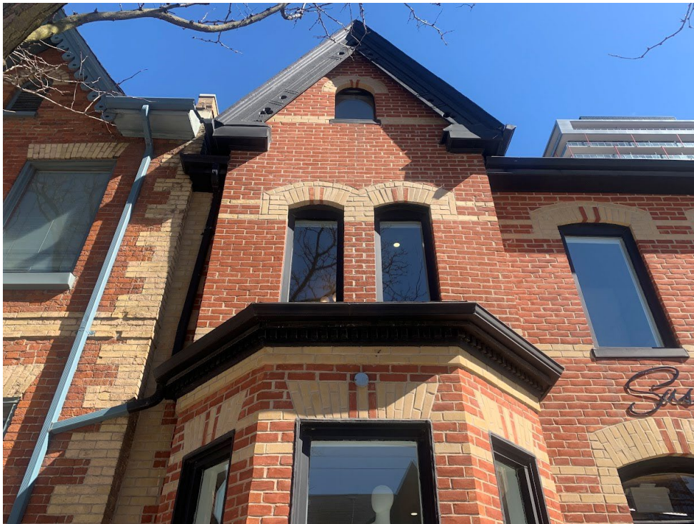
Figure 6. Current photo showing the decorative brickwork and wood detailing on north bay at 111 Berkeley Street and the south edge of 115 Berkeley Street at left (Heritage Planning, 2024)
