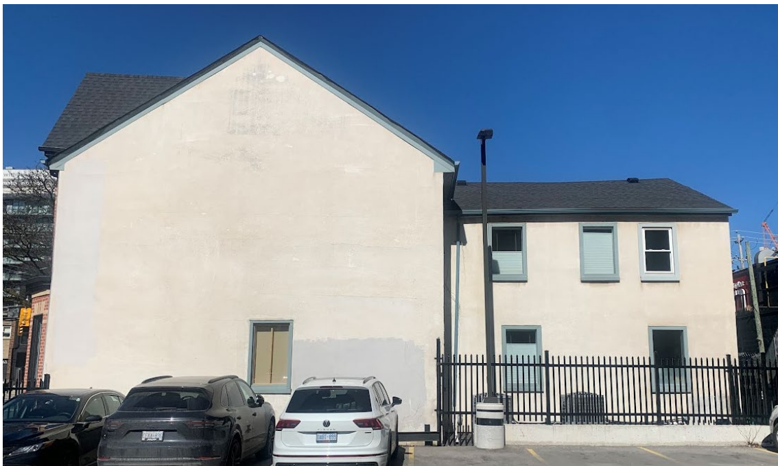
Figure 5. South elevation of the property at 111 Berkeley Street, showing the rear wing at right (Heritage Planning, 2024)
