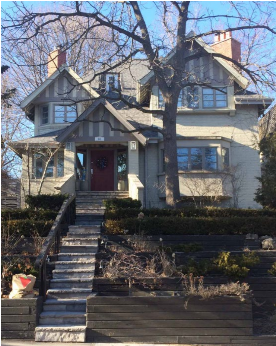
Figure 2. View of the primary (south elevation) of the property at 64 Woodlawn Avenue West in 2018 (Heritage Planning, 2018)
