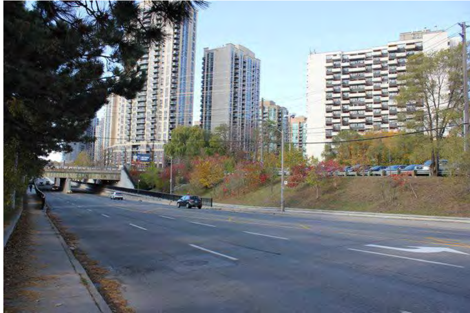
Bloor at Rail Overpass
