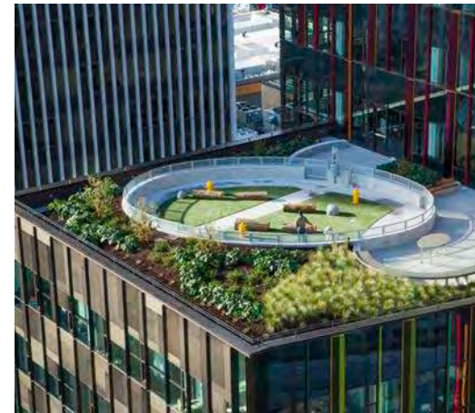
Rooftop Dog Park, Amazon Doppler Building, Seattle
