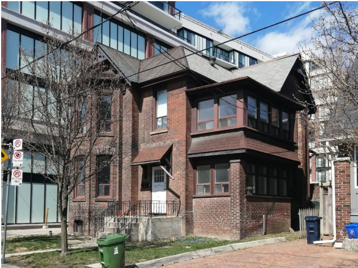
View of south and east elevations at 26 Millwood Road showing c.1926 two-storey enclosed porch (Heritage Planning, 2024).
