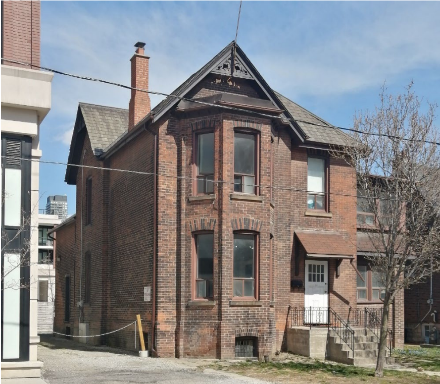
View of south and west elevations at 26 Millwood Road showing two-storey three-sided bay, brick voussoirs, stone sills and decorative gable pediments (Heritage Planning, 2024).
