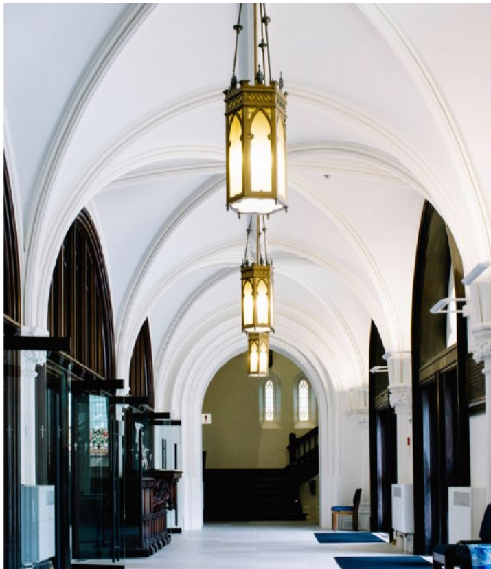
Figure 20 Narthex showing pointed arch openings and vaulted ceiling looking north towards stairwell annex featuring finely carved staircase (Knox, 2019).
