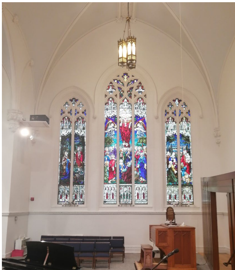
Figure 17 South transept showing vaulted-arch ceiling and tripartite pointed-arch stained-glass windows with wooden tracery (Heritage Planning, 2024).
