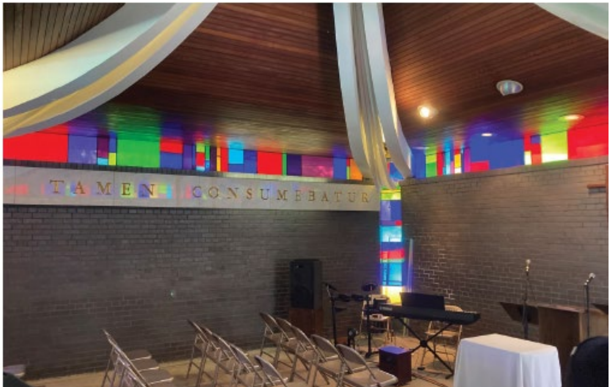
Figure 29 Interior of Chapel showing dark brick cladding, and horizontal ribbon windows fitted with coloured glass, wood panelled ceiling and exposed curved steel beams (Heritage Planning, 2024).
