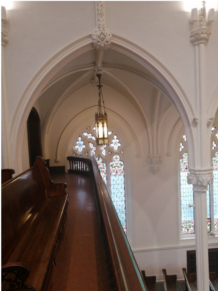
Figure 19 Section of south aisle showing decorative plasterwork including vaults, strapwork, capitols and drip moulds (Heritage Planning, 2024).
