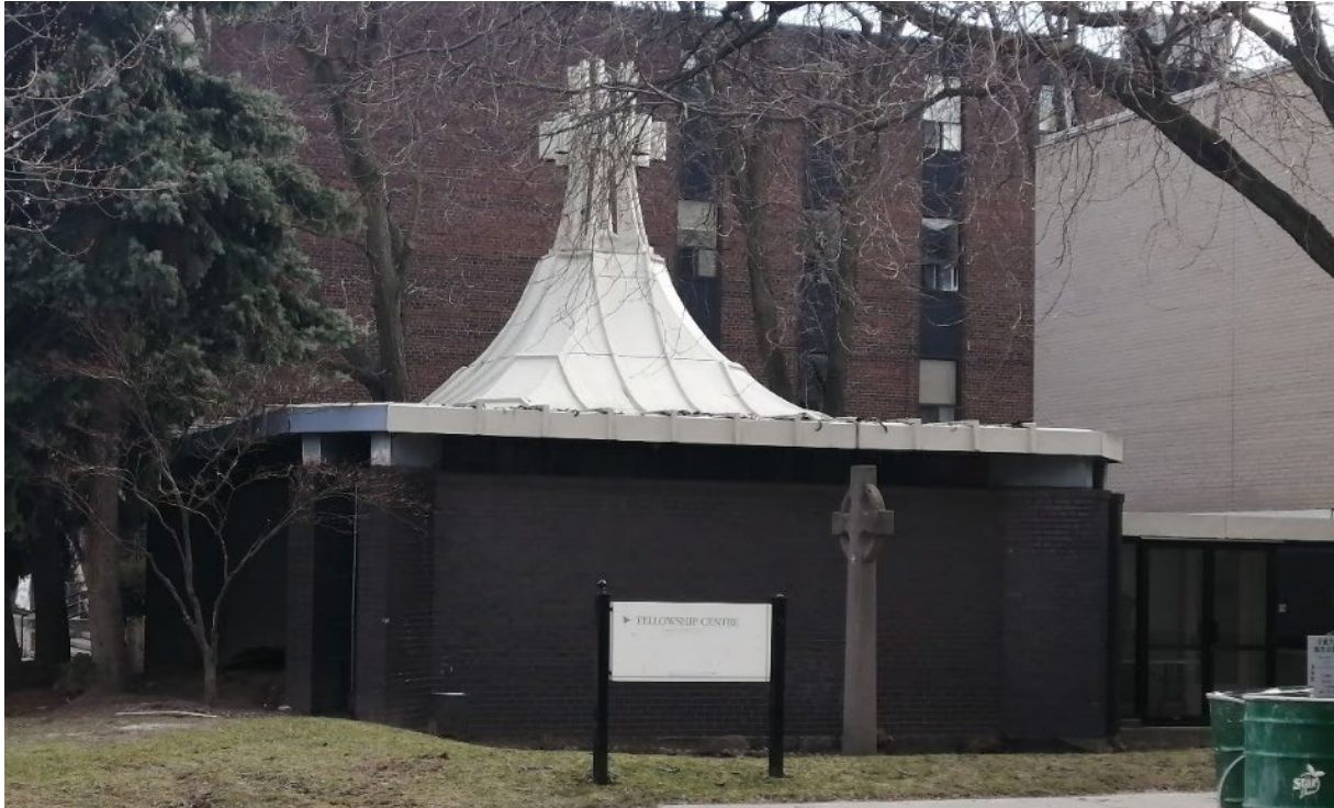
Figure 27 Southwest view of Chapel featuring corner buttresses, dark brick cladding, and curved metal roof. The 1961 Cross is in the foreground (Heritage Planning, 2024).
