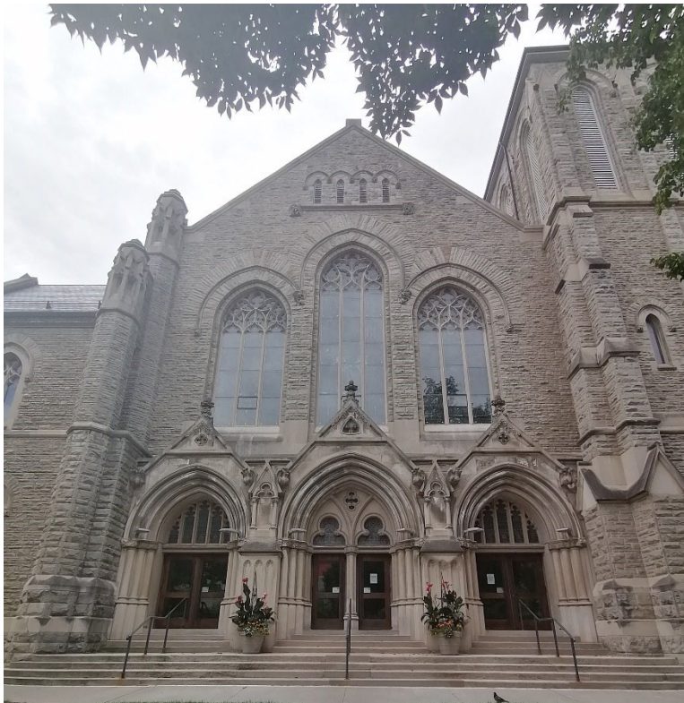
Figure 3 Detail of central section of principal (east) elevation showing triple entrance with pointed arch openings featuring carved stone colonnettes, archivolts, tracery, and gables with gargoyles, quatrefoils, and finials (Heritage Planning, 2024).
