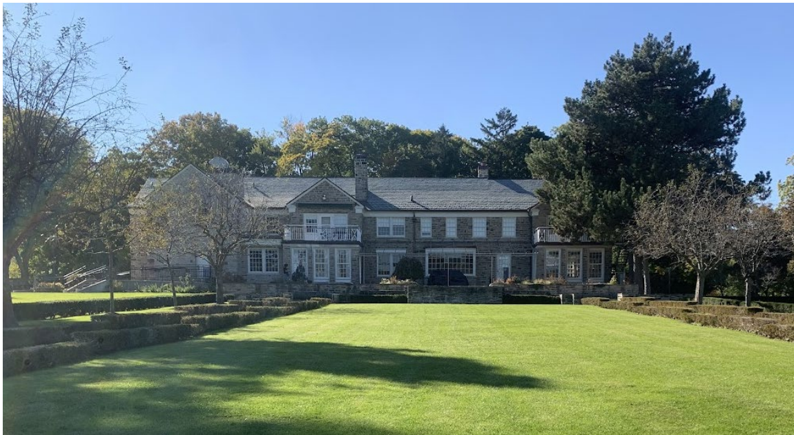
Image 14: The Main House, rear (east) elevation, from the east end of the formal terraced gardens (Heritage Planning, 2024)
