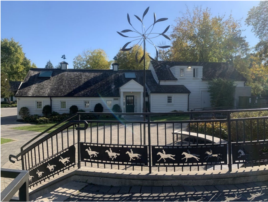
Image 27: 2012 circular stair and ramp with Muybridge horse detailing in the railings (Heritage Planning, 2024)
