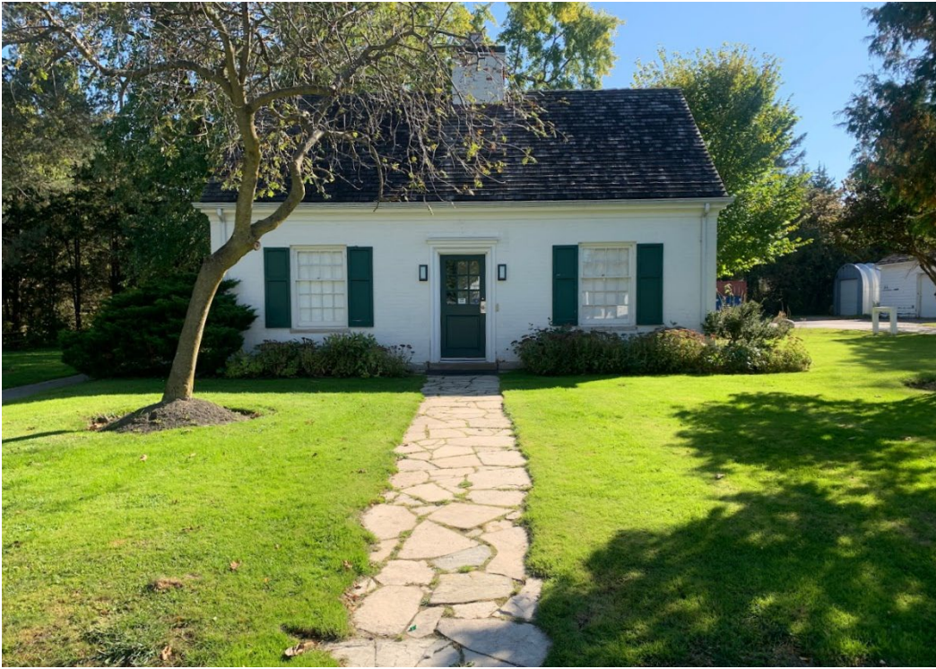
Image 21: Cottage D, principal (north) elevation (Heritage Planning, 2024)
