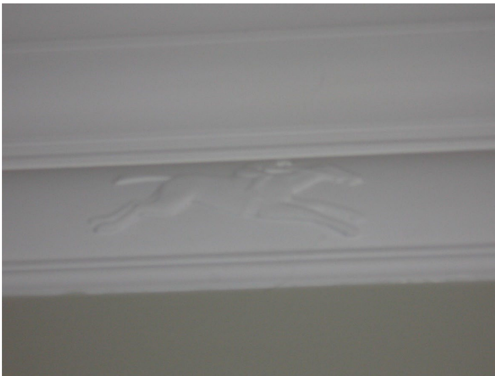
Image 15: Detail of the Muybridge horse plaster frieze on the second-floor landing in the Main House (Heritage Planning, 2010)
