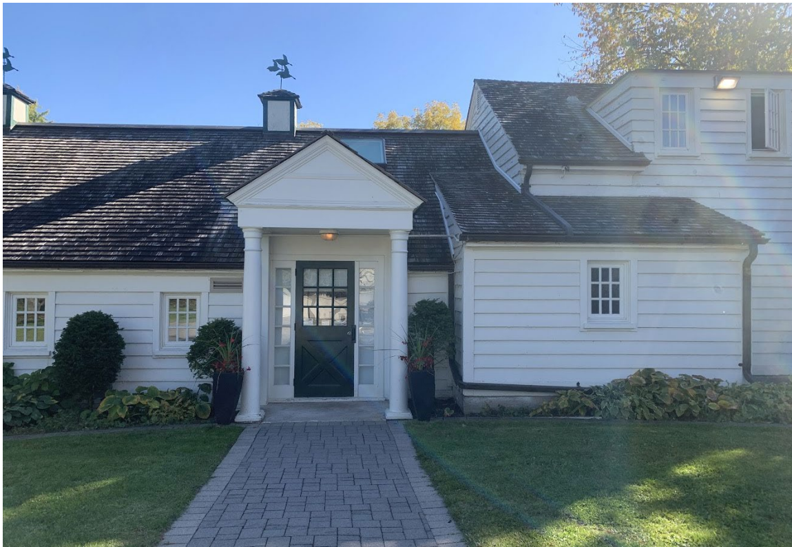
Image 17: The Stables, north (principal) elevation (Heritage Planning, 2024)
