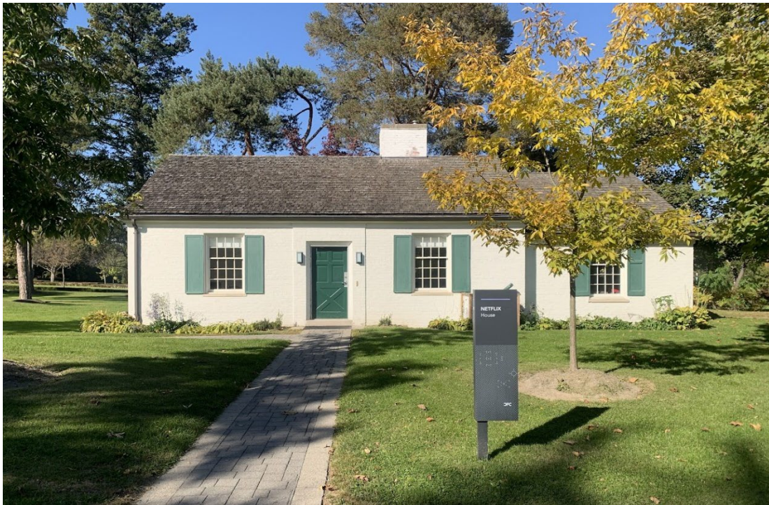
Image 19: Cottage C, principal (south) elevation (Heritage Planning, 2024)
