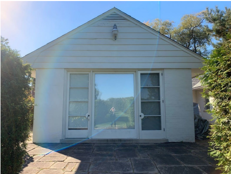
Image 26: The Gatehouse, east elevation, showing E.P. Taylor's office picture window and opening onto a flagstone terrace. As seen in the reflection, the opening was intended to provide a distant view across the open grounds toward the east end of the property. (Heritage Planning, 2024)
