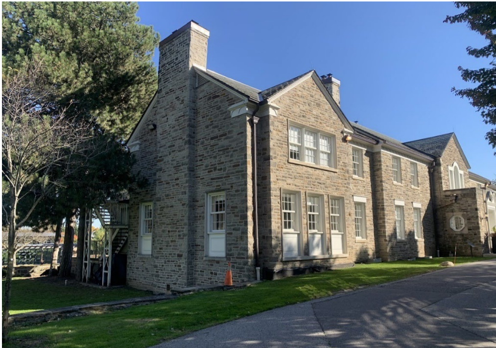
Image 13: Main House, looking southeast and showing the 1948 north wing by Earle C. Morgan (Heritage Planning, 2024)
