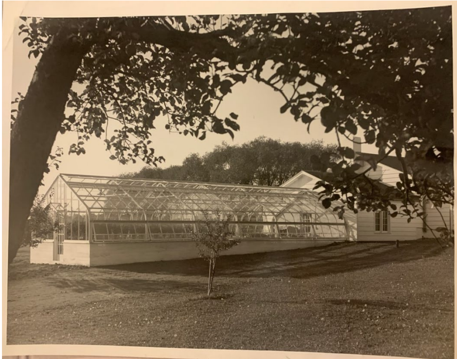
Image 7: 1950s Archival photo of the Potting Shed & Greenhouse with the Lord & Burnham greenhouse structure with curvilinear glazing (Archives of Ontario)
