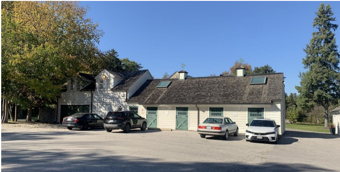
Image 18: The Stables, rear (south) elevation, showing the four horse stall doors and integrated double car garage. (Heritage Planning, 2024)
