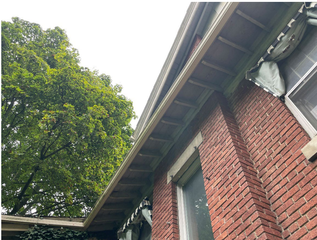
Figure 12: detail view showing an example of the open eaves with wooden tongue-and-groove soffits and exposed rafters, 2024 (City of Toronto Heritage Planning)
