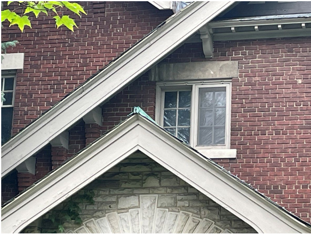
Figure 9: detail view showing an example of the brick corbelling and stone brackets below the eaves and the gable overhang detailing, 2024 (City of Toronto Heritage Planning)
