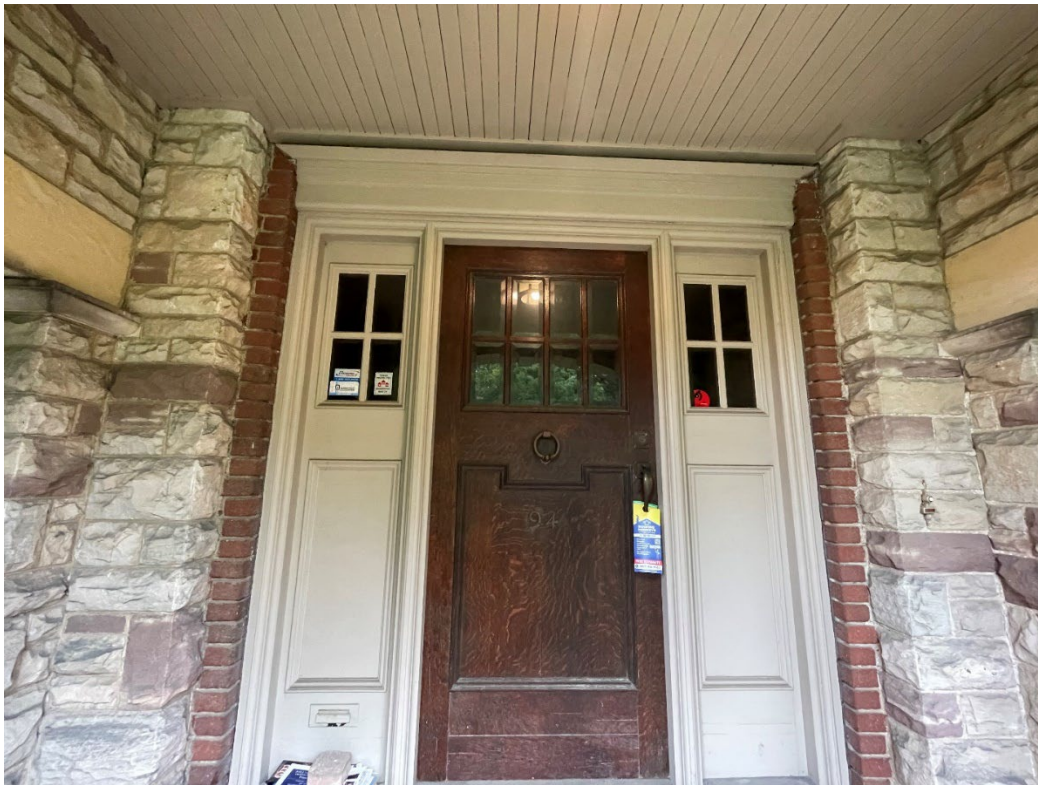
Figure 11: the main entrance (west façade) and doorway assembly and porch stonework detailing and wooden tongue-and-groove ceiling, 2024 (City of Toronto Heritage Planning)
