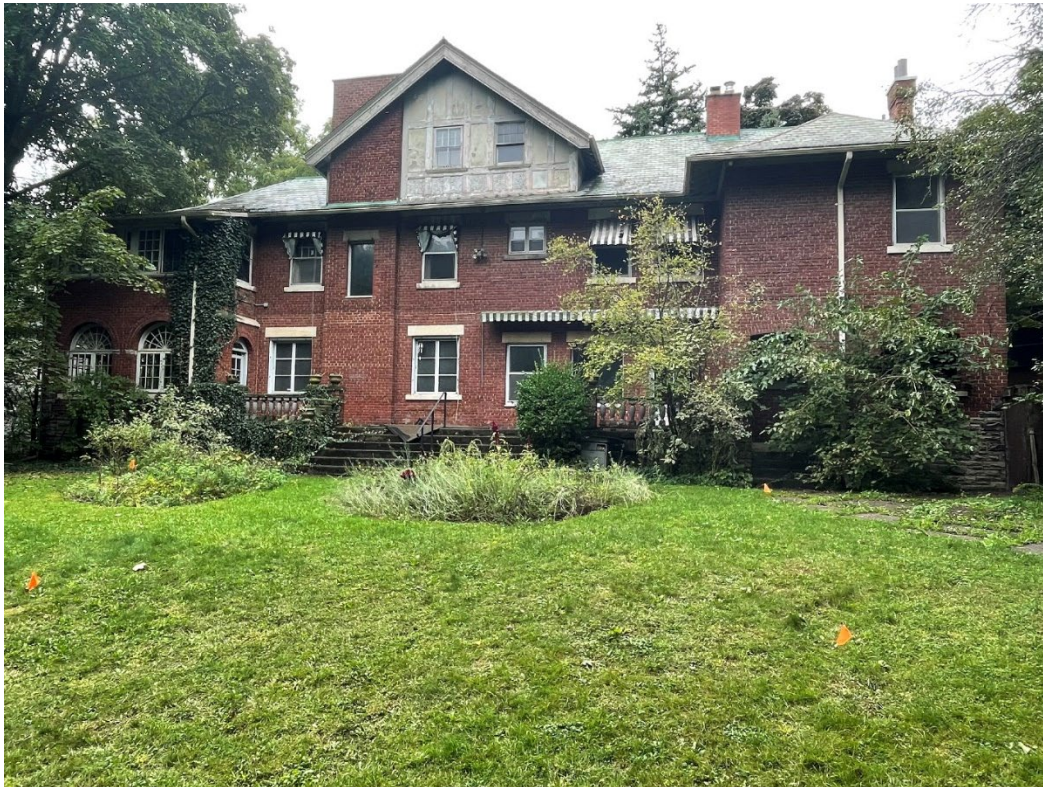
Figure 4: rear (east) façade, 2024 (City of Toronto Heritage Planning)
