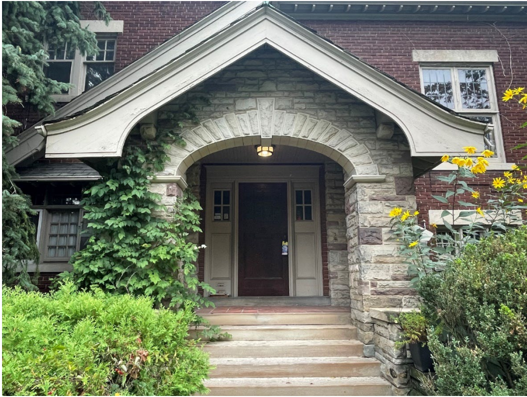
Figure 10: the front porch on the main (west) facade, 2024 (City of Toronto Heritage Planning)
