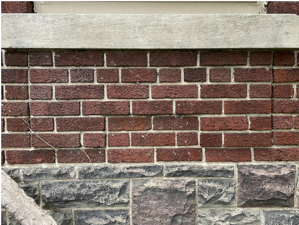
Figure 7: detail view showing the apron brickwork below window; also the rough-dressed stonework detailing and an example of a smoothly dressed window sill, 2024 (City of Toronto Heritage Planning)
