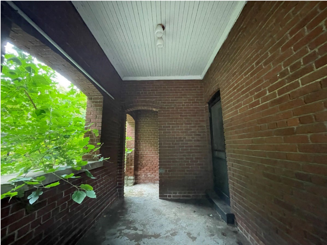
Figure 16: rear, open, integral porch with wooden tongue-and-groove ceiling, 2024 (City of Toronto Heritage Planning)
