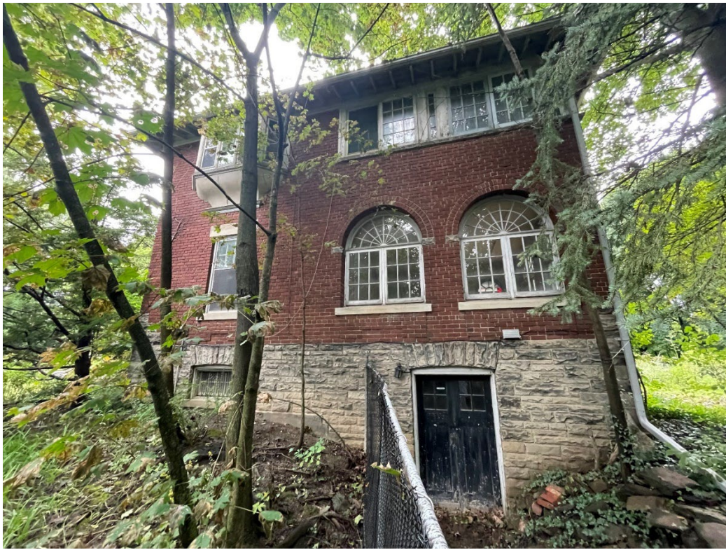
Figure 5: side (south) façade - note the cantilevered Jacobethan window on left side of second storey - 2024 (City of Toronto Heritage Planning)
