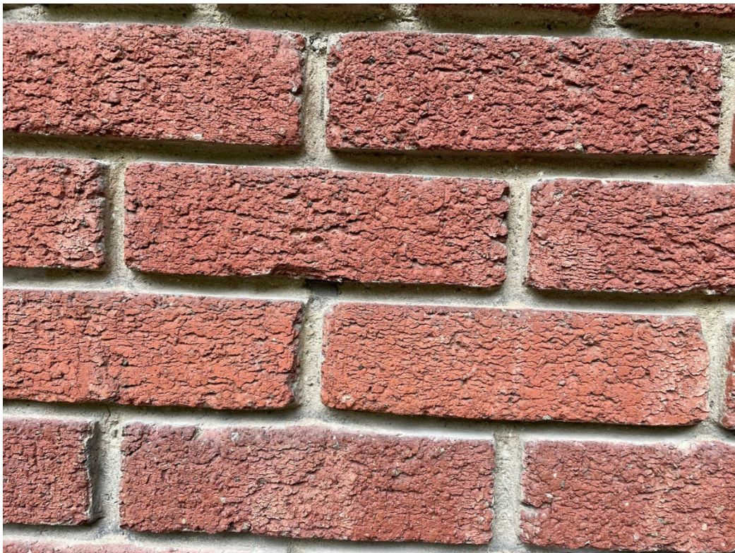
Figure 8: detail view showing the rustic red brick cladding with wide, deeply recessed mortar joints, 2024 (City of Toronto Heritage Planning)
