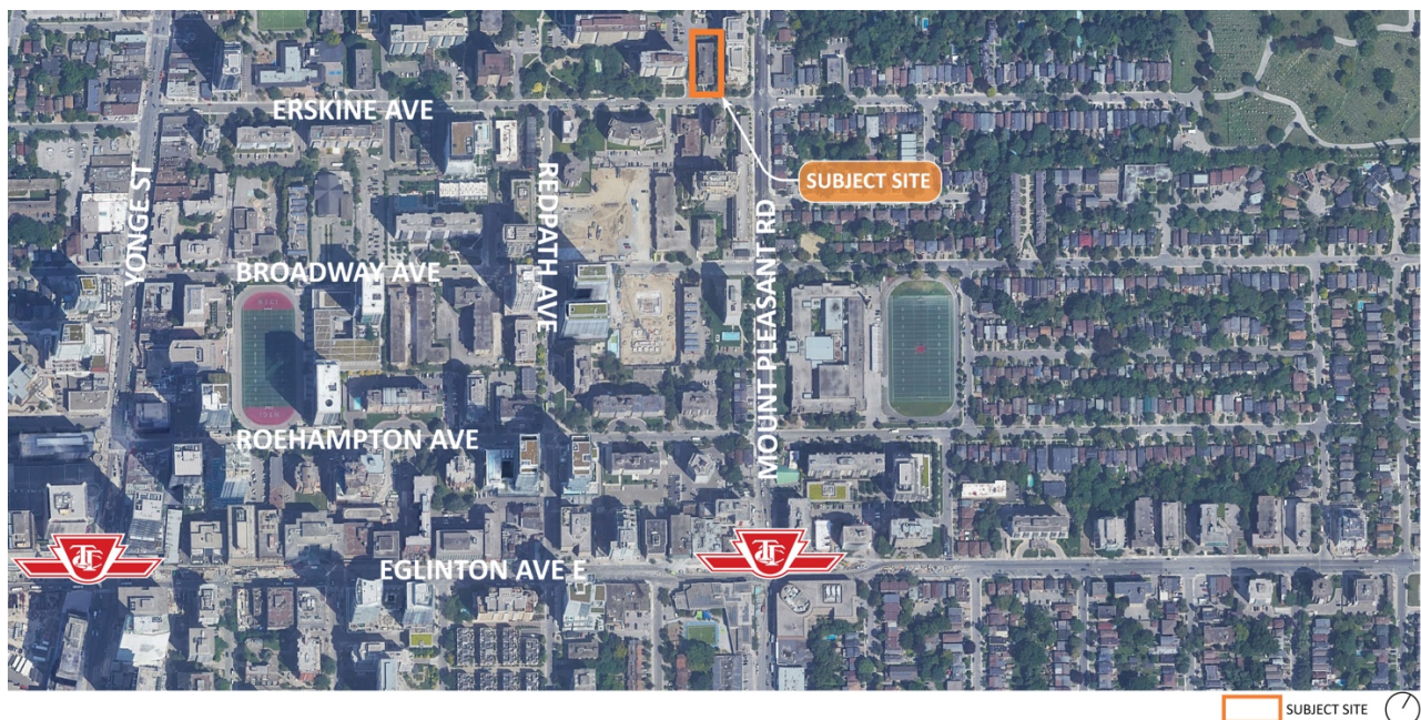
Figure 1: Aerial View of the Subject Site.
