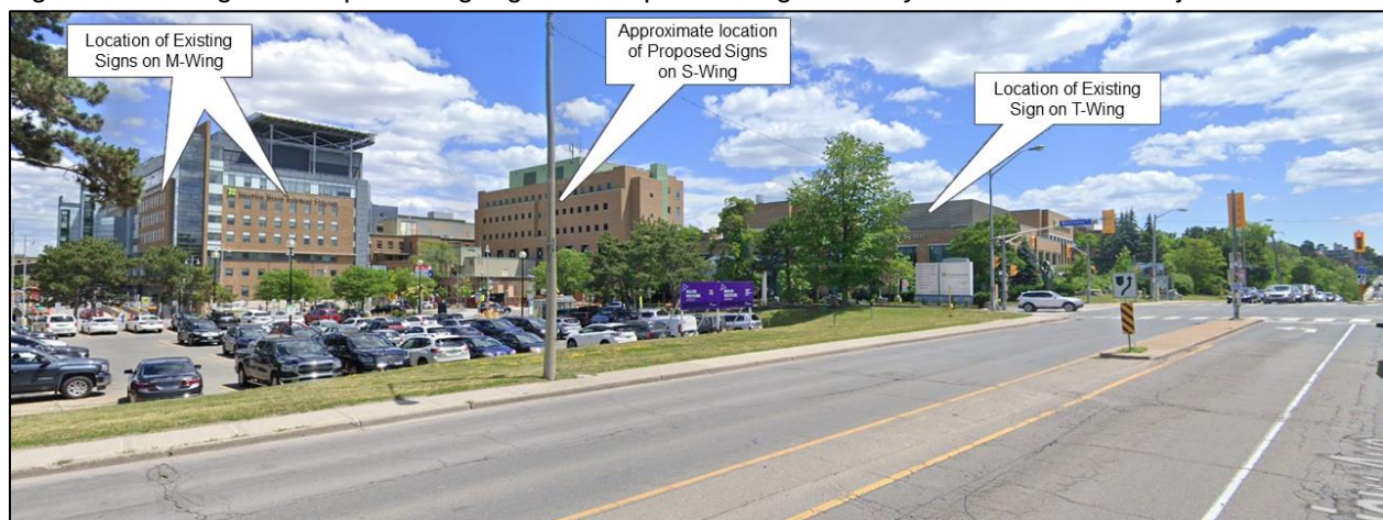
Figure 8: Existing and Proposed Signage on campus looking from Bayview Ave to the Subject Premises
