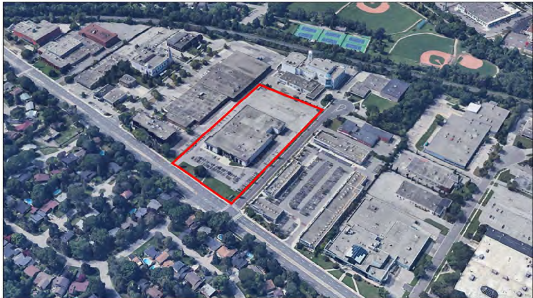
FIGURE 2: 3-D AERIAL OF SUBJECT SITE (OUTLINED IN RED); VIEW FROM THE NORTHEAST
